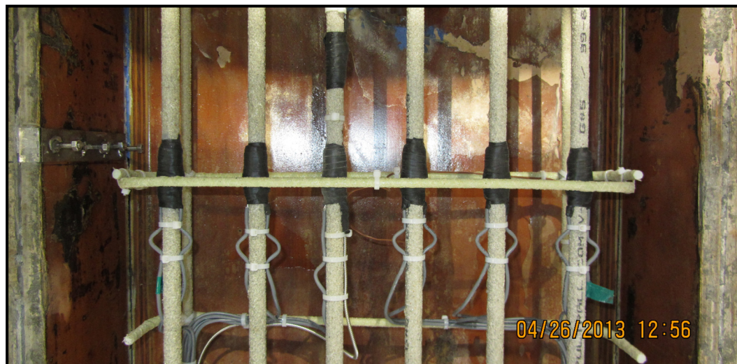
Figure 3-23 Strain Gauges and FOS in Formwork
