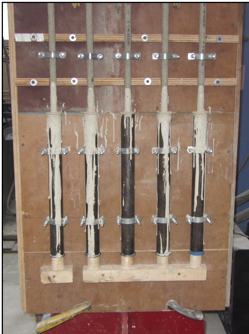
Figure 3-13 Anchor Installation on GFRP
