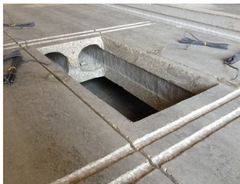
Figure 3.6: Typical CFRP Groove Layout Around Opening
