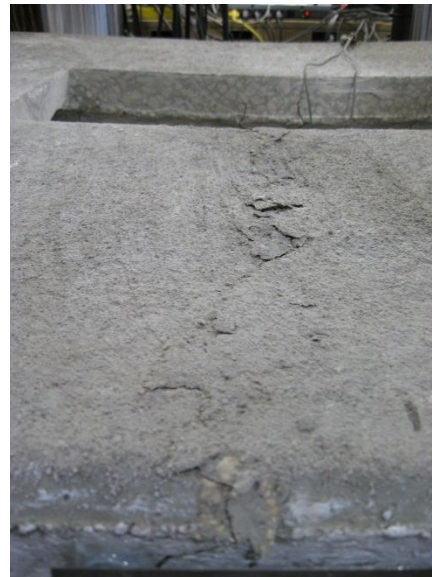
Figure G.8: II-1-S0-FO Specimen at Failure
