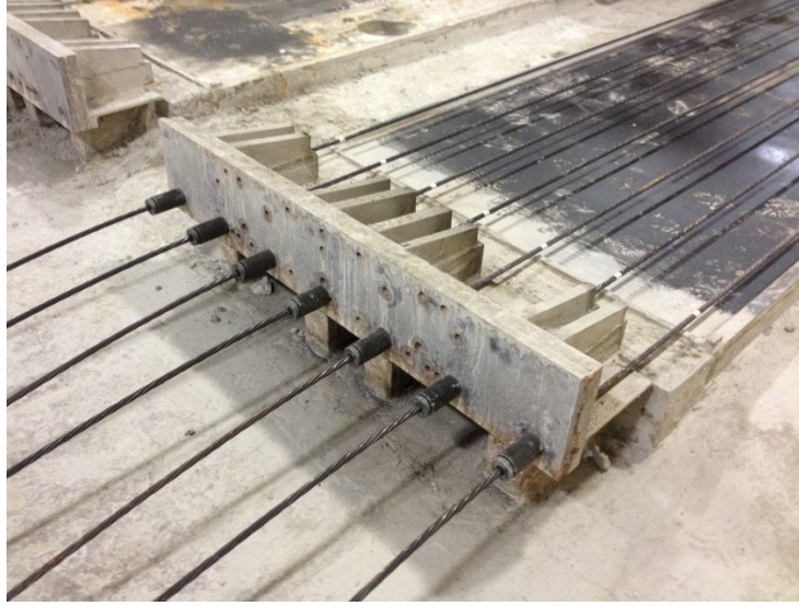
Figure 3.20: Anchor and Prestressing Tendon Setup
