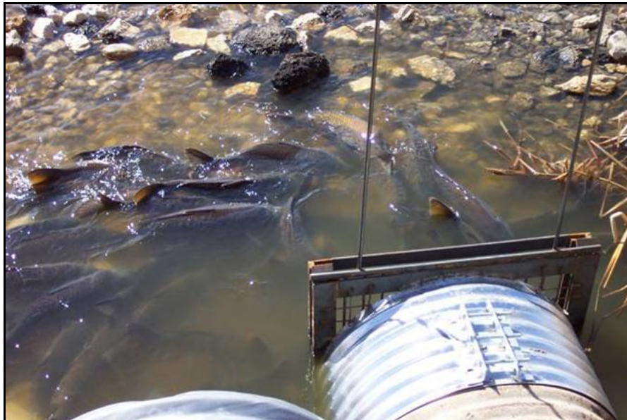
Figure 2-4. Group of large common carp at culverts, forming a biological barrier, potentially blocking entrance by other fish into Mid-Blind Channel (Photo by Candace Parks).
