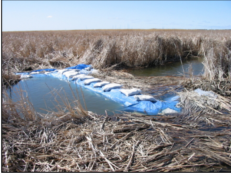
Figure 1-10. Sandbag dike constructed on May 2, 2002 at the channel entrance of Mad Woman Bay, to isolate the pond from Section 5 Bay and the main marsh (Photo by Dale Wrubleski).
