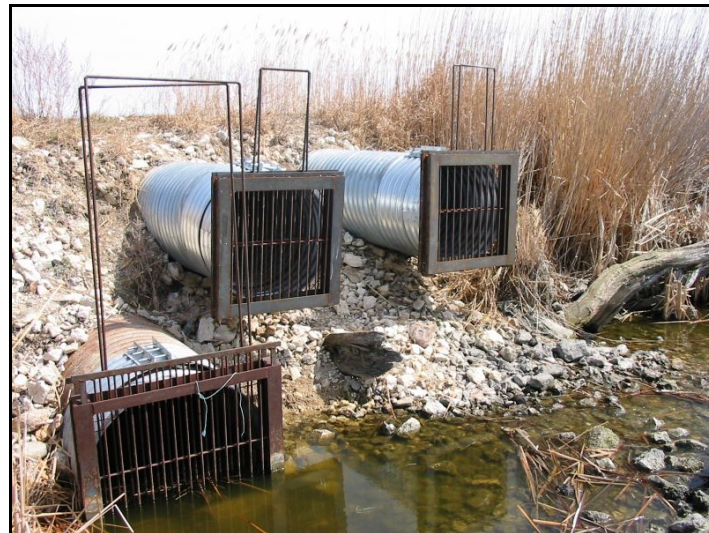
Figure 1-7. Three screened culvert covers under the Delta Marsh Field Station winter road prevented large common carp from entering Mid-Blind Channel from West Blind Channel (Photo by Dale Wrubleski).
