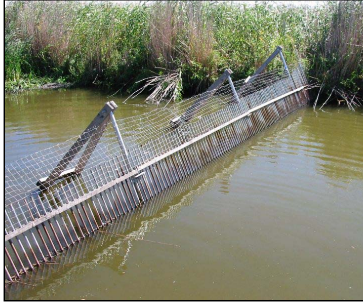
Figure 1-6. Conduit fence constructed in channel upstream of Section 5 Bay on April 22, 2002. Stucco fencing was added to the top of the conduit fence to prevent fish like common carp from leaping over during periods of wind set-up (Photo by Dale Wrubleski).
