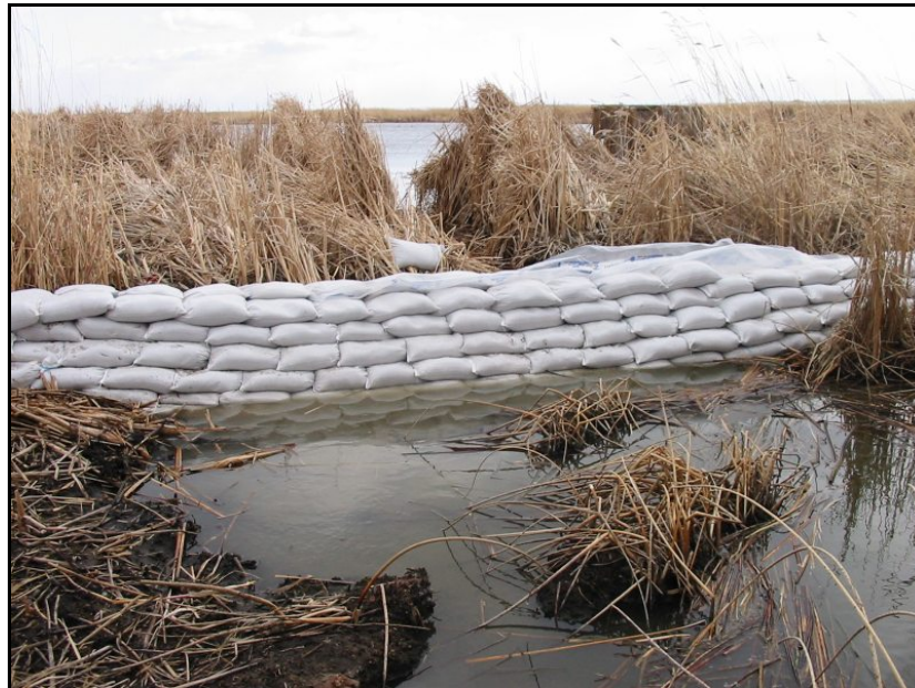
Figure 1-9. Sandbag dike constructed at entrance of South Pitblado's Channel on April 24, 2002 (Photo by Dale Wrubleski).
