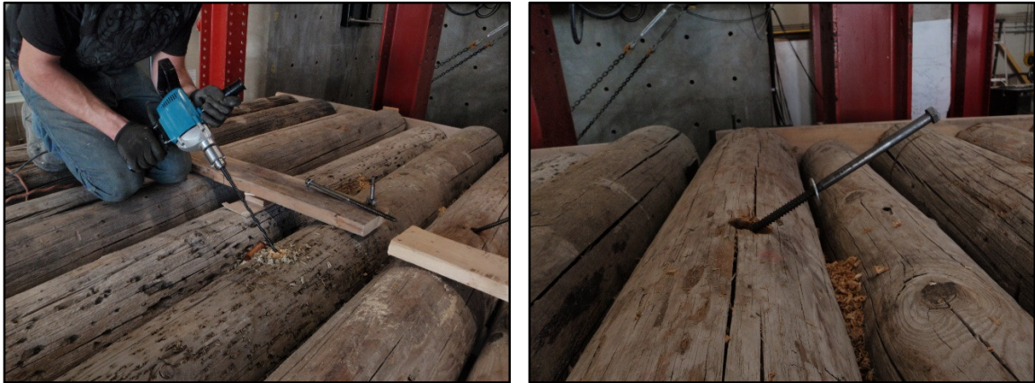
Figure 3-17. Installation of lag screws to connect panels.
