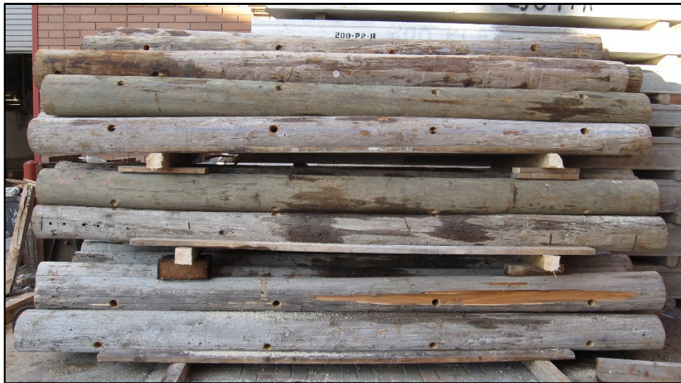
Figure 3-13. Logs for the anchored log deck with holes drilled at four locations.
