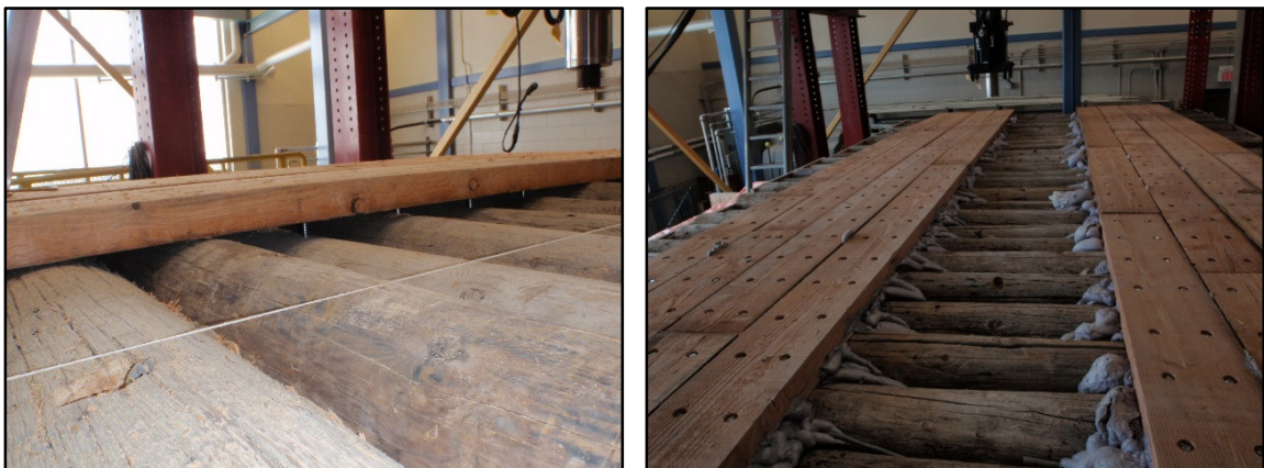
Figure 3-18. Gaps under wearing planks and high density foam.
