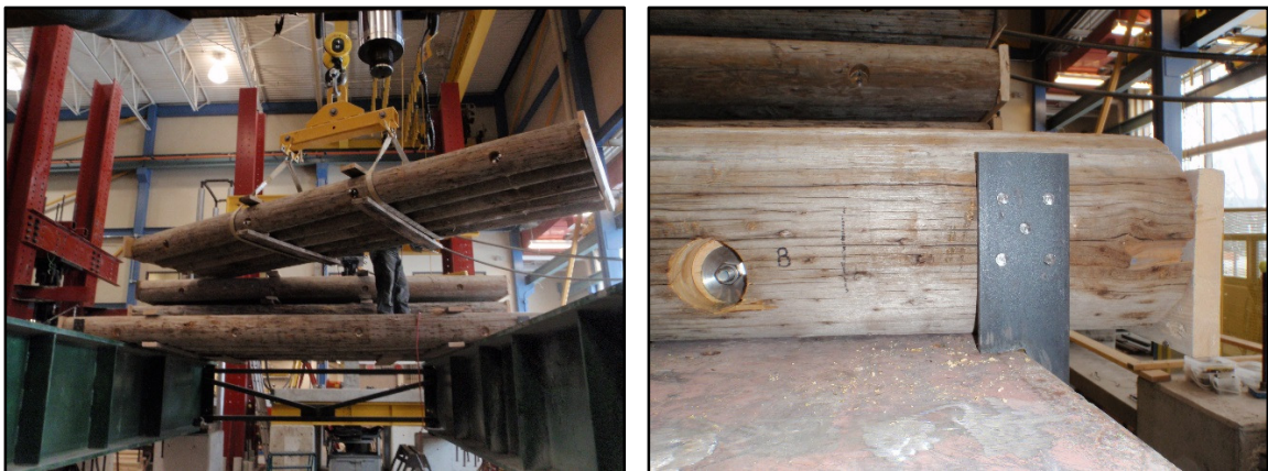
Figure 3-16. Placement of panels on girders and steel clip angle.
