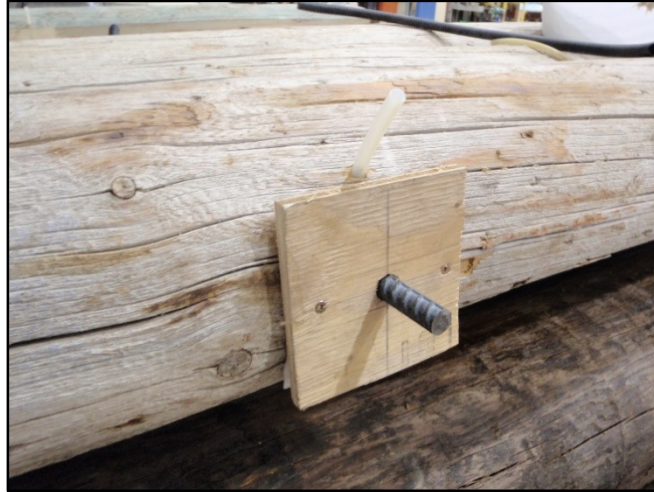
Figure 3-6. Steel reinforcing bar and grout tube.
