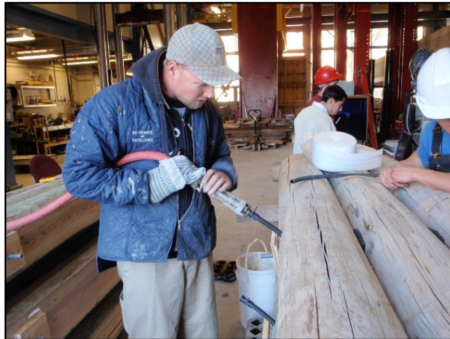
Figure 3-7. Grouting of log panels.
