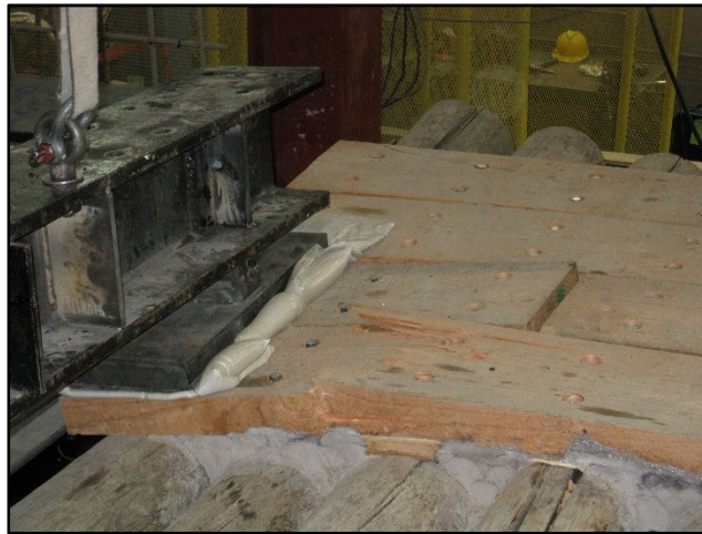
Figure 4-6. Failure of wearing plank.
