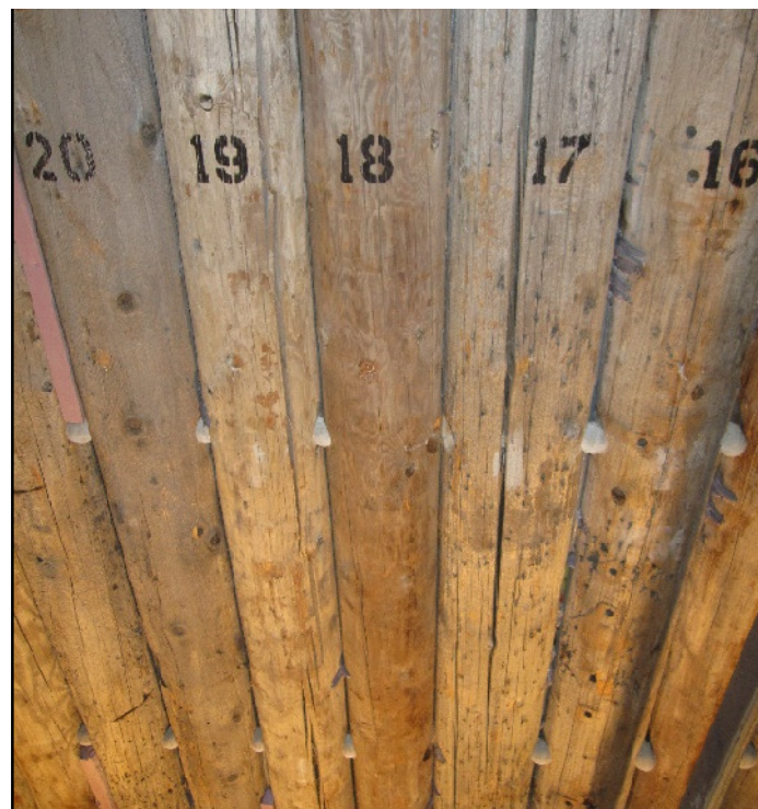
Figure 4-14. View of underside of logs after static test.
