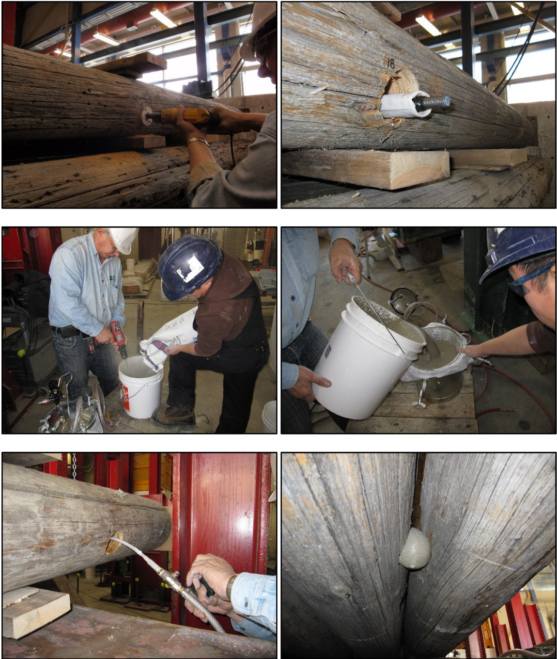
Figure 3-15. Grouting of Cintec anchors.
