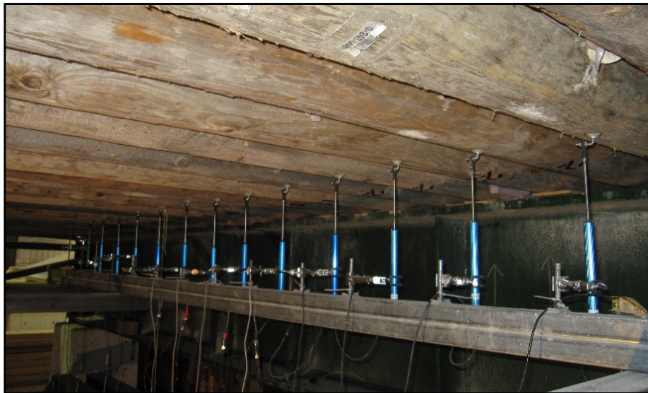
Figure 4-10. LVDTs located underneath the deck.
