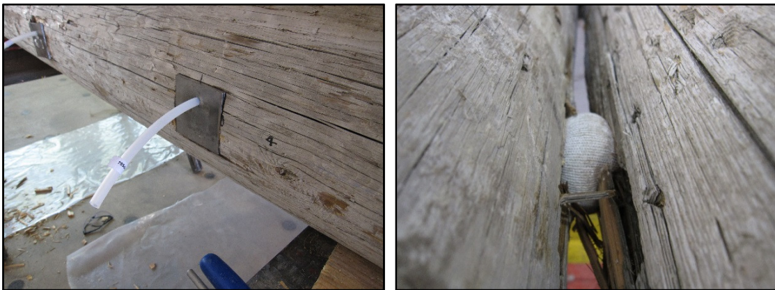
Figure 3-9. Cintec anchor installed in log panel and expansion of sock with grout.
