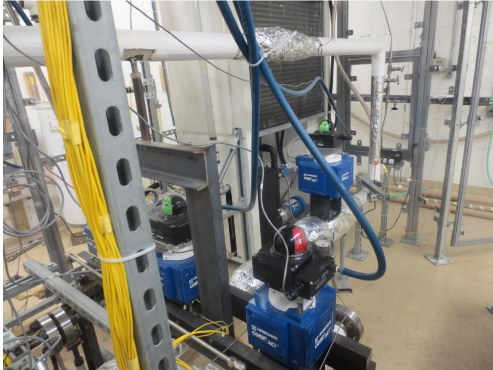
Figure D.4: Hot side of natural circulation loop
