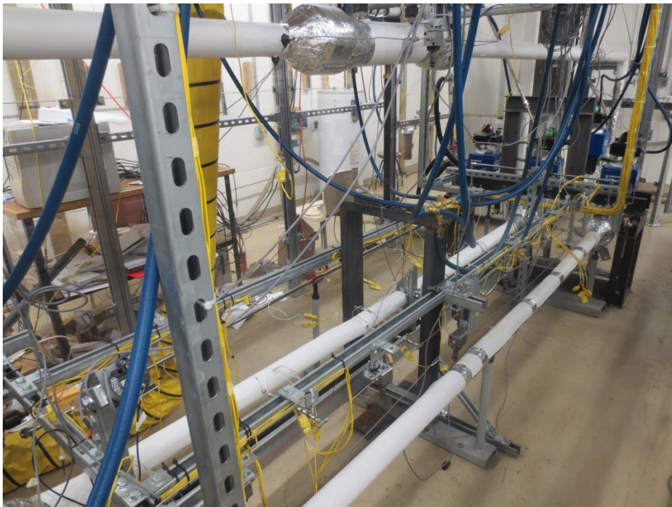
Figure D.3: Heated section (middle channel) and the heat exchanger
