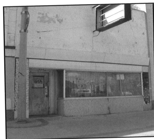
Figure 25: An example of the lack of care that inhabits many of the buildings along Main Street.
