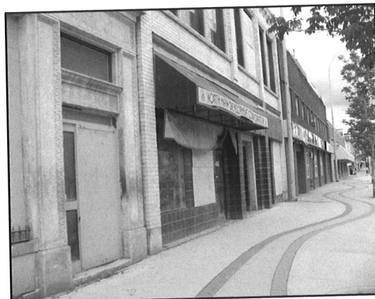
Figure 24: Many buildings along Main Street appear to be vacant.
