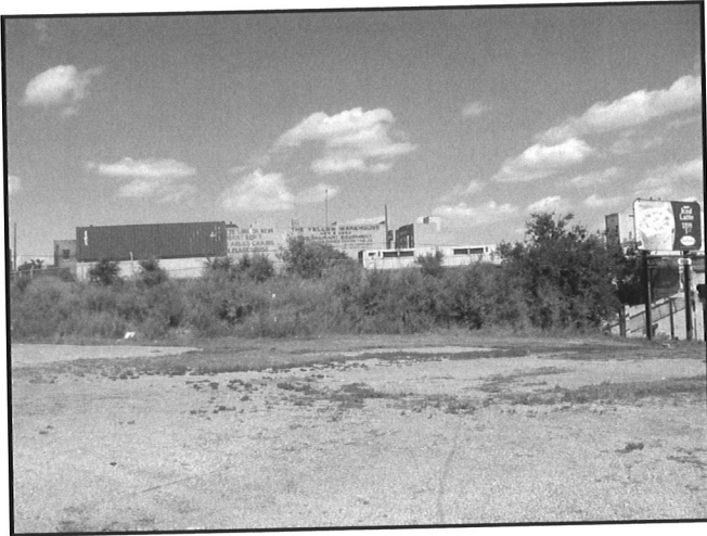
North view of the railway embankment.
