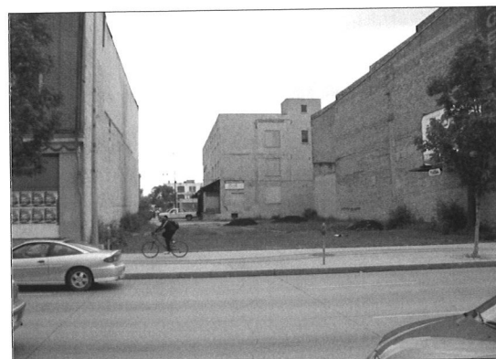
Figure 3: ‘Missing Teeth’: A void between buildings
