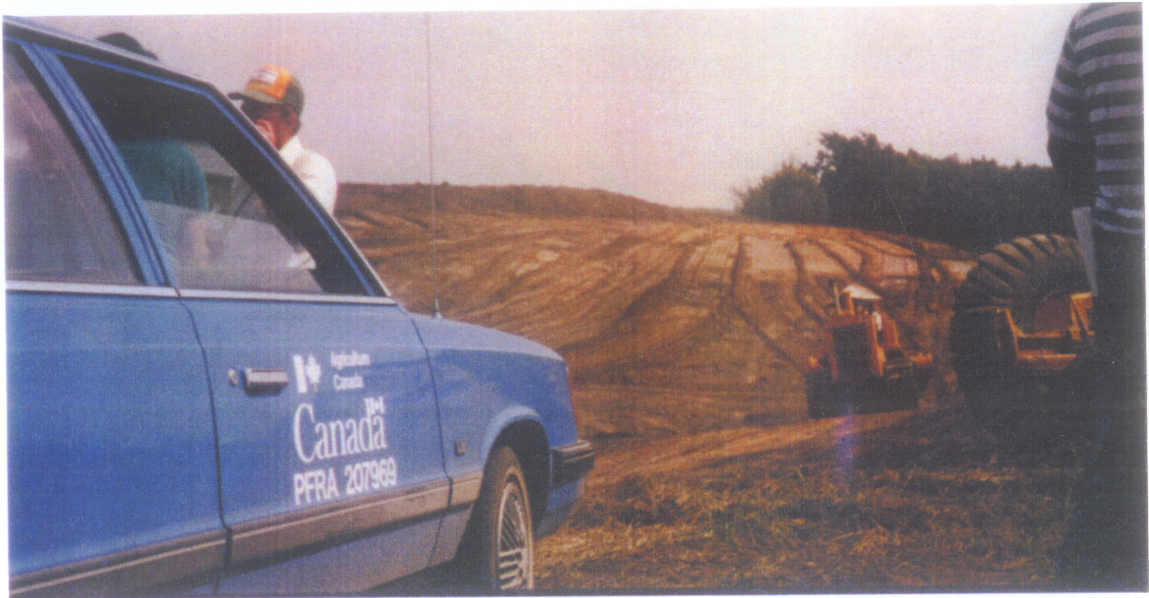
Plate 4c Typical Dry Dam Under Construction in Deerwood Region Source: Bryan Osborne
