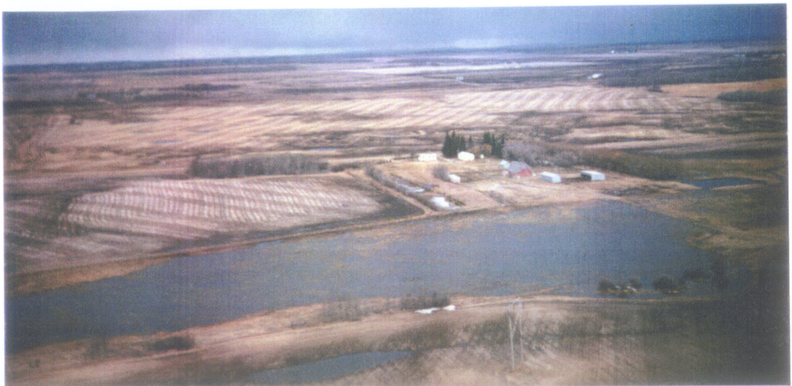
Plate 4d Typical Backflow Dam in Deerwood Region Source: Bryan Osborne
