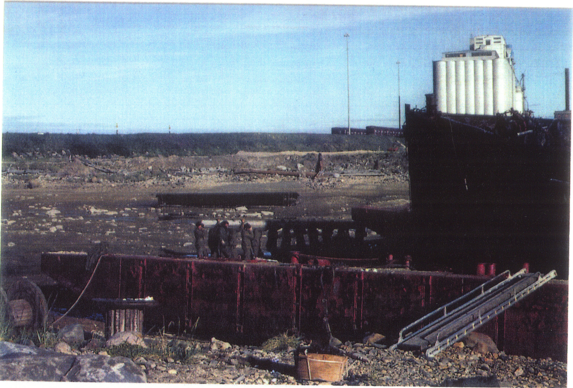
Figure 4a. Position of floats surrounding vessel.
