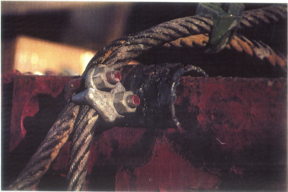
Figure 5b. Modification to floats designed to reduce cable abrasion.
