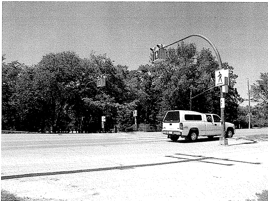
Figure 23. Existing pedestrian crossing at Henderson Highway and Bunn's Creek Greenway
