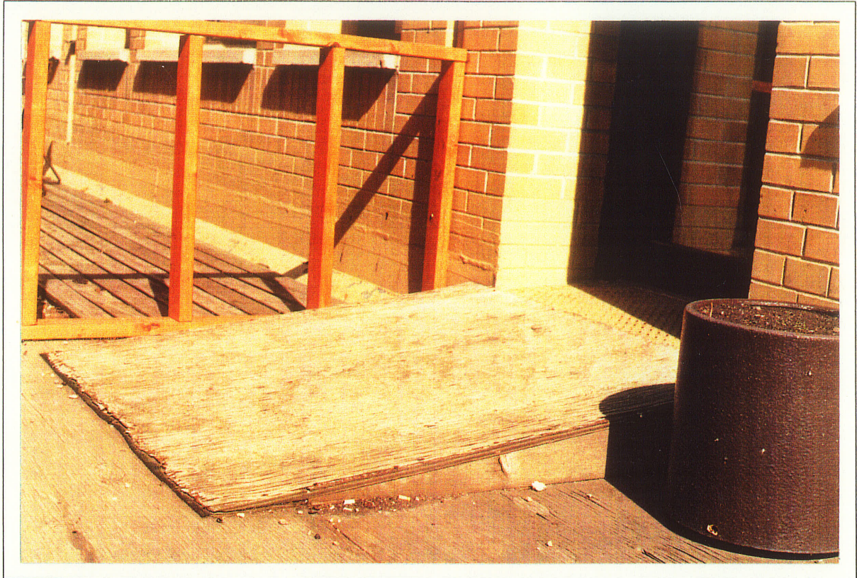
Figure 8. Examples of poor detailing and deteriorating condition.
