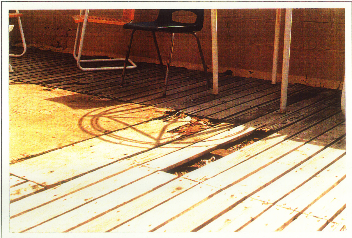
Figure 9. The wood decking is rotting away.
