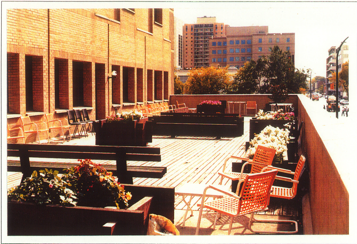
Figure 7. Second floor roofdeck looking south.
