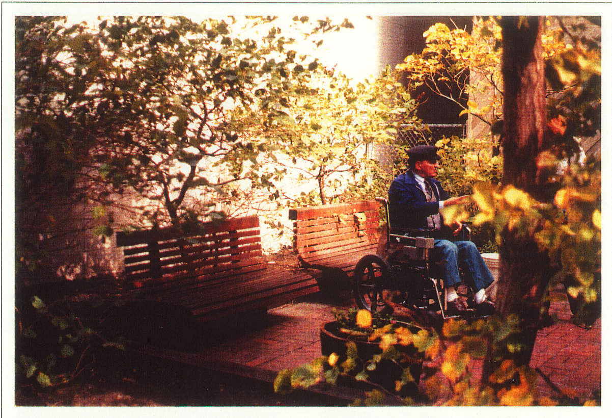
Figure 6. Settling of benches has lowered the seat heights beyond comfortable use.
