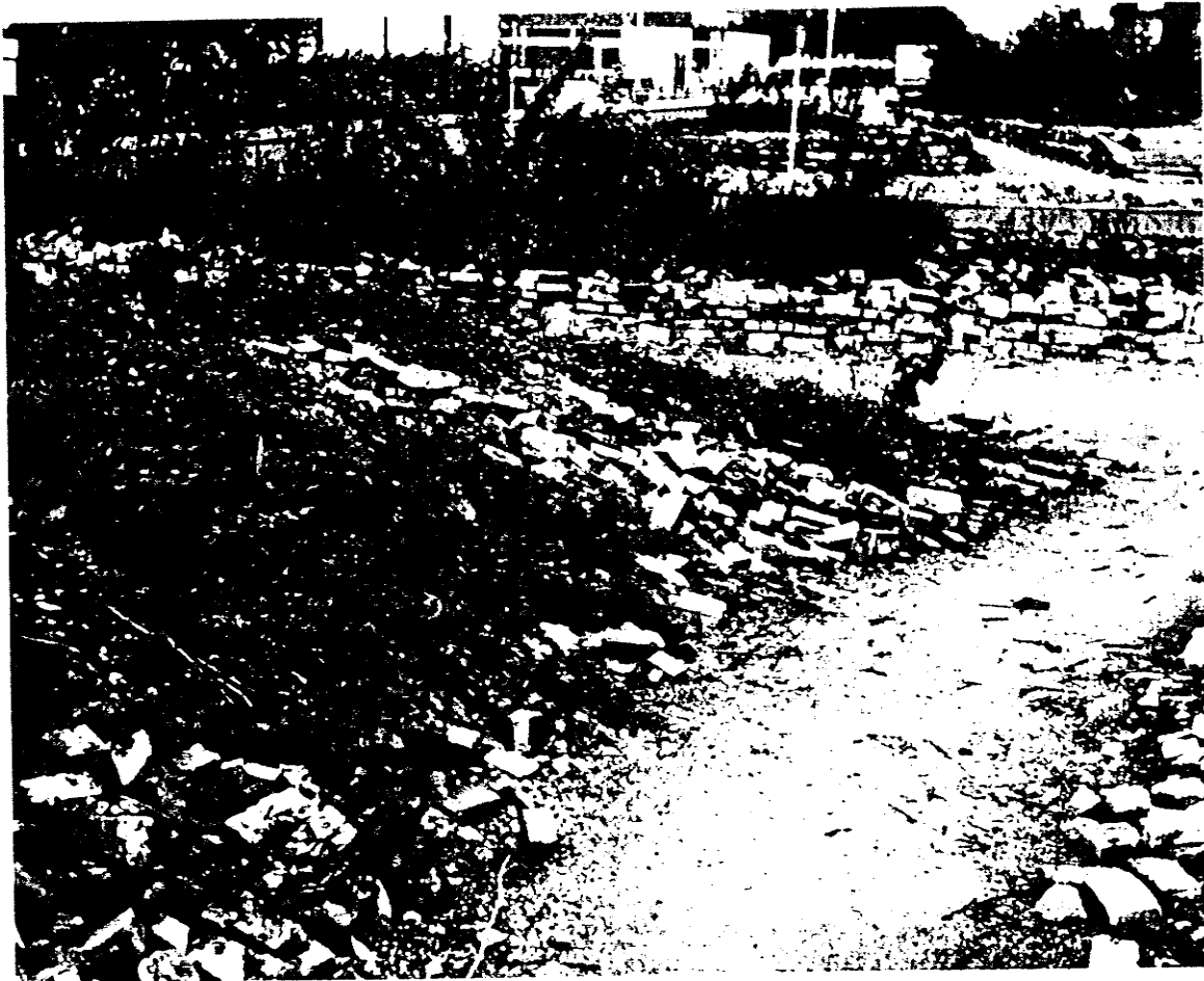
FIGURE 8: TERRACING USING BUILDING RUBBLE AT KENNEDYLAAN, HERRENVEEN, IN HOLLAND. 31
