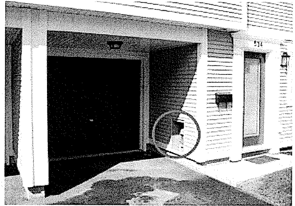
Figure 24: Service elements are integrated into the design of this building.
