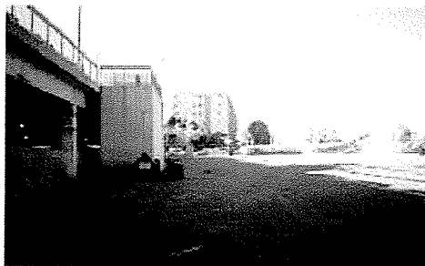
East end of site (Zellers Parking Garage and North Parking Structure)
