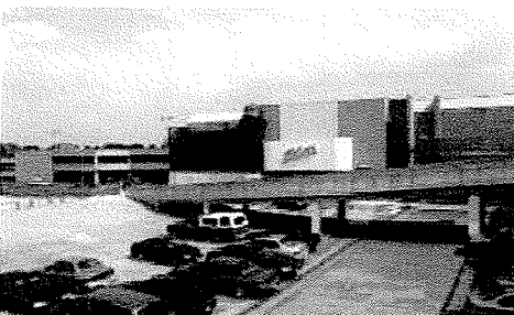
North-east corner of site (Zellers Parking Garage and North Parking Structure 2nd level)
