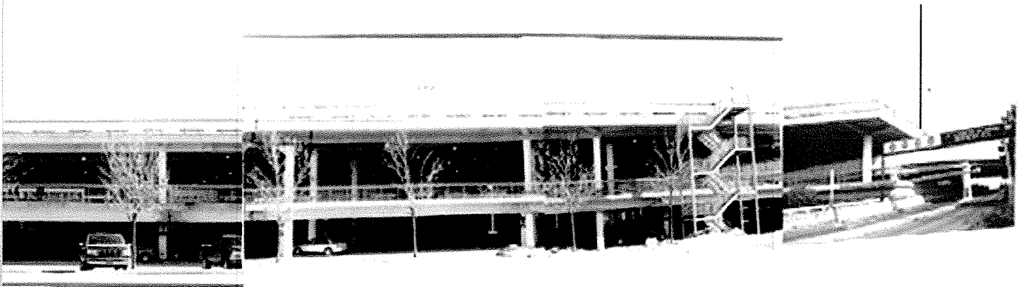
access ramp (from Woodridge Cres.)
