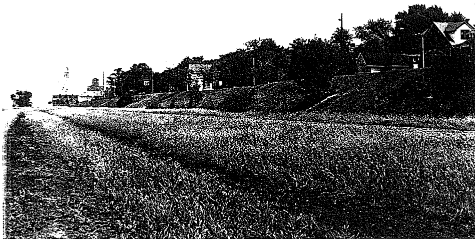
Figure 4.25: View of original beach ridge at the eastern end of the site
