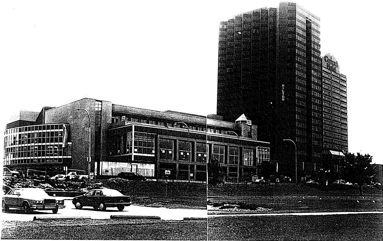
Figure 4.5: Renovated Cleary Auditorium and Convention Centre (left) and the two completed riverfront hotels (the Hilton and the Compri)
