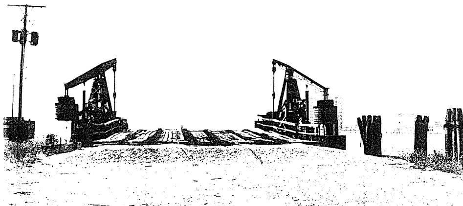
Figure 4.22: Barge ferry dock and leveling apparatus
