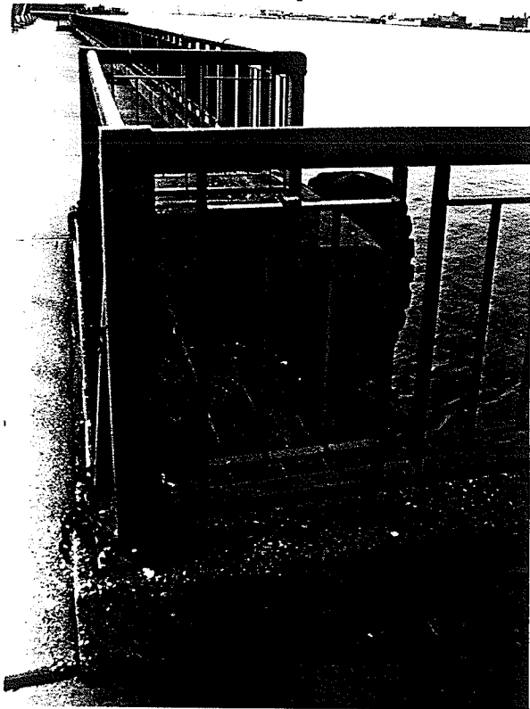
Figure 4.31: Railing along the promenade in Dieppe Gardens
