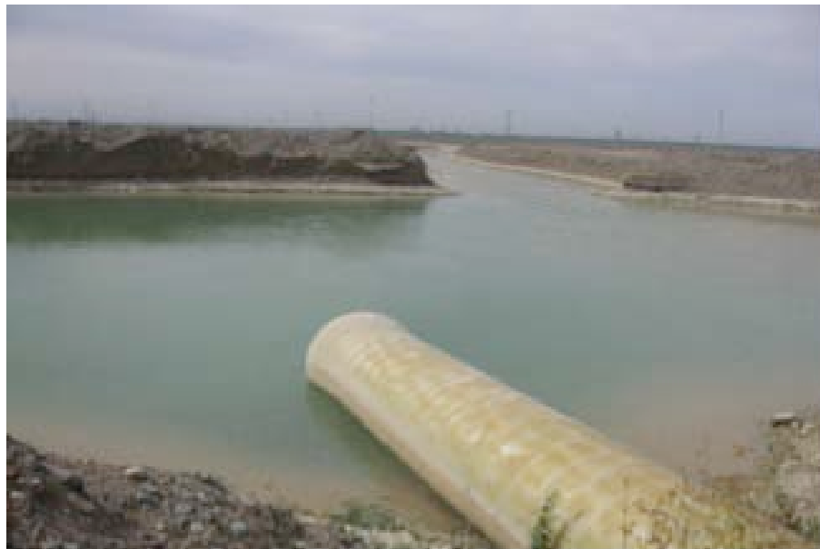
Photo 9 Wastewater from purification process directly discharged into an empty land
