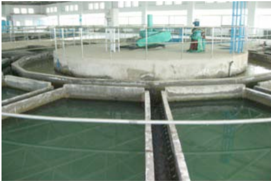
Photo 6 Mechanical stirring process in No.3 WPP
