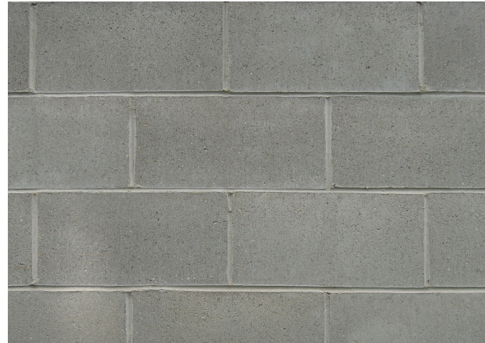
FIGURE 77 - EXISTING CONCRETE MASONRY UNIT WALL
