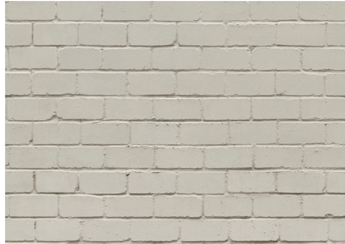
FIGURE 76 - EXISTING PAINTED BRICK WALL
