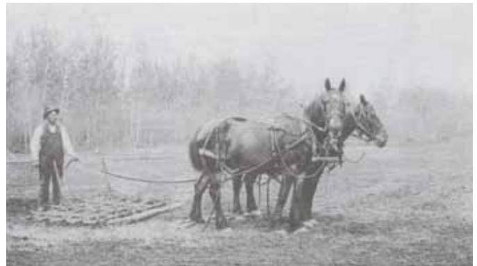
Figure 2.4: Grading of Windsor Park Golf Course
