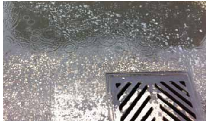
Figure 2.5: Storm-water contaminants entering a sewer.
