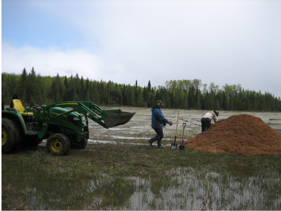
Figure 3.3. Pile of wood chips amendment and equipment used to move amendments around site.
