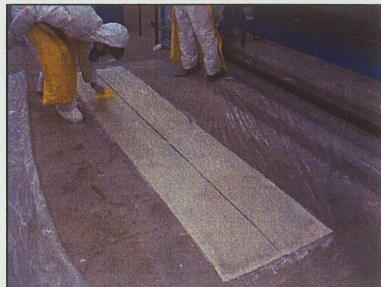
Figure 4-10 Preparing unidirectional glass fiber woven sheet
