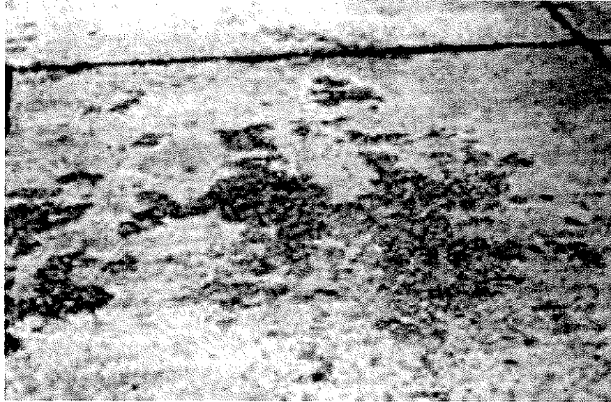
Figure 2.2: Concrete Scaling Caused by Freeze-Thaw Cycles in the Presence of Deicing Chemicals (Adopted from Portland Cement Association)
