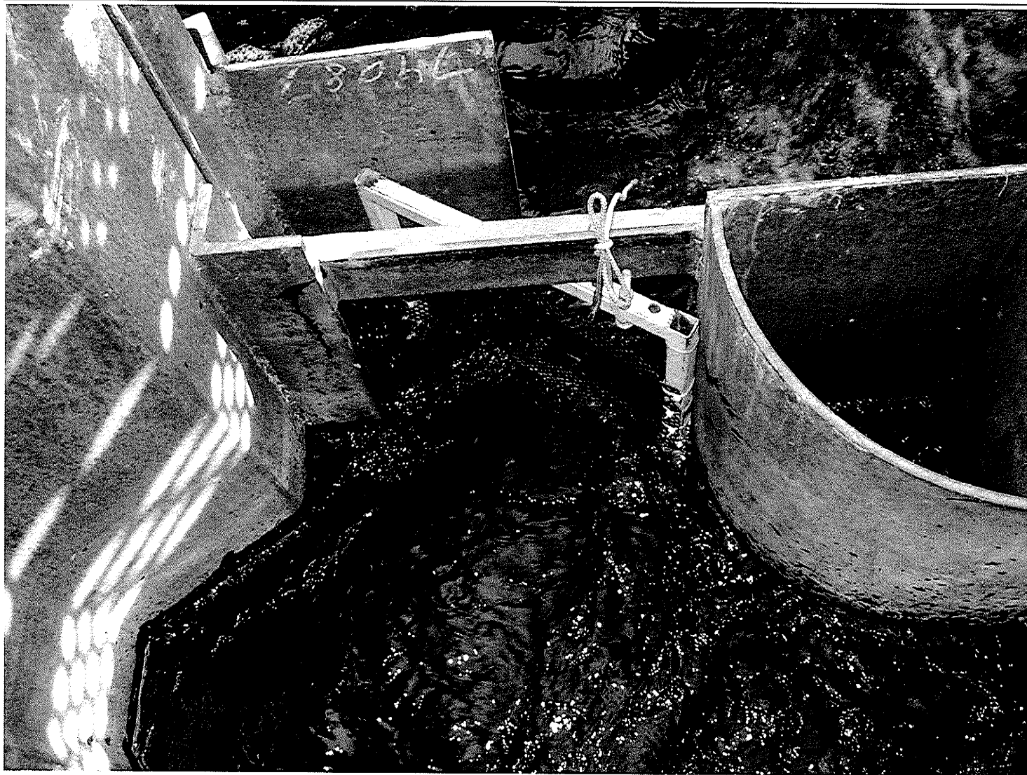
Figure 3. Placement of screen at exit of 9 th chamber in the Rocky Creek fishway.
