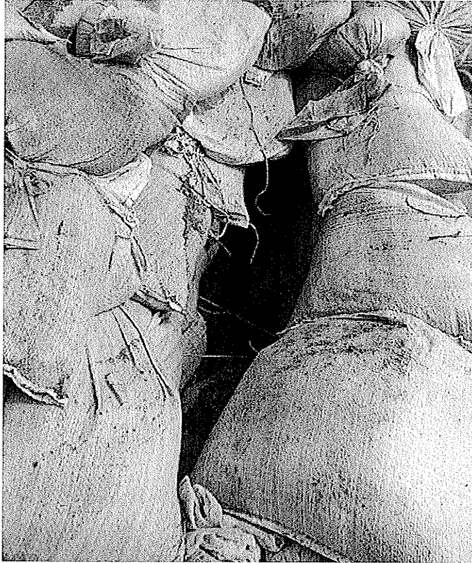
Figure 5.9 – Gap Between Sandbags Observed During Exhumation of Dike A2.
