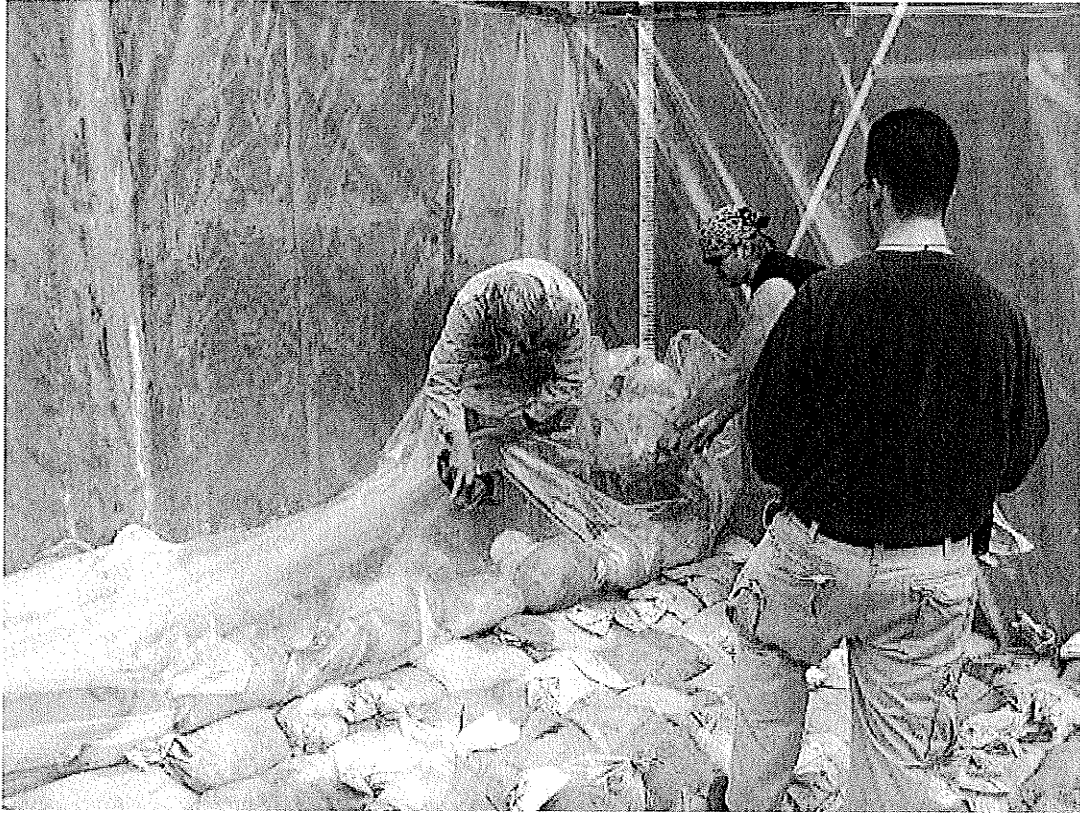
Figure 5.72 – Volunteers Weaving PES into Dike E, View to the North-east.
