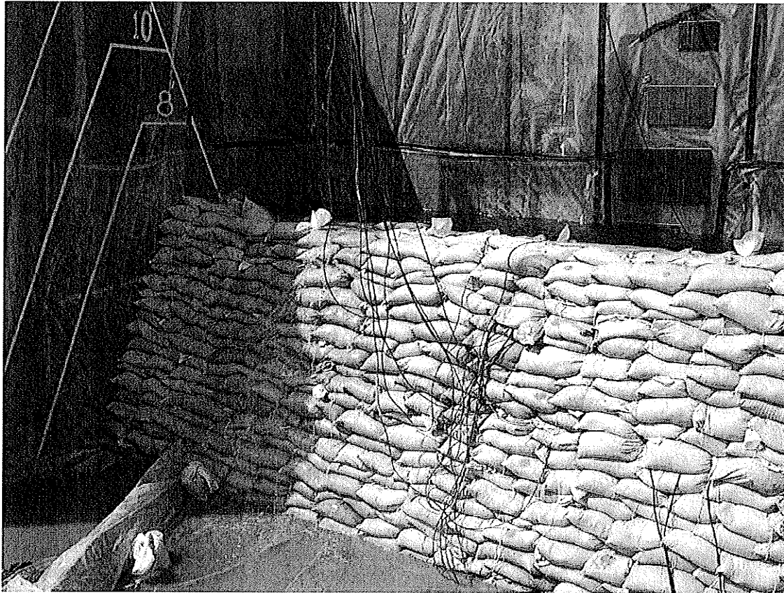
Figure 5.41 – Dike C2 During Overtopping Loading, View to the North-west.
