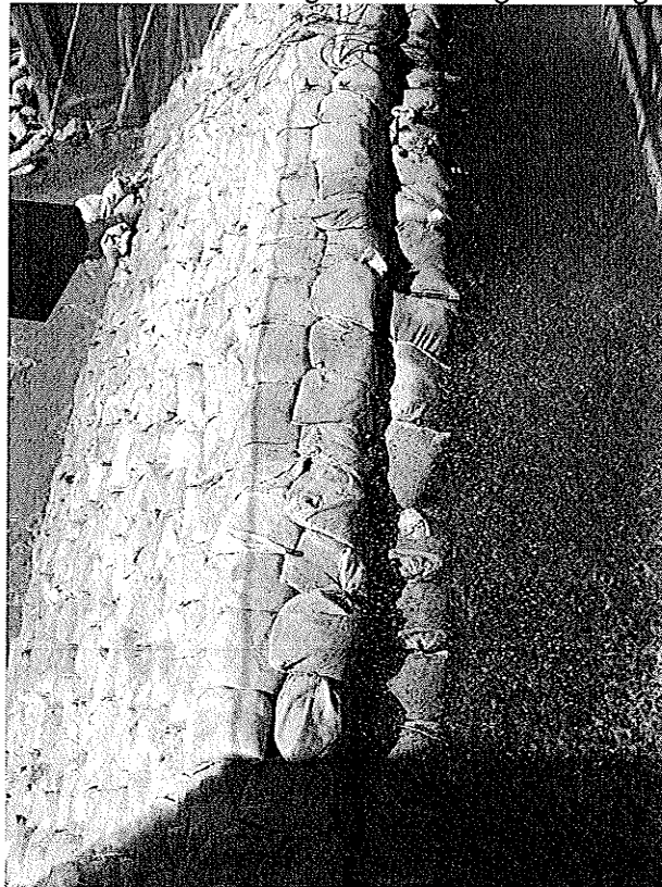
Figure 5.61 – Dike D2 during Above Design Loading, View from Above.
