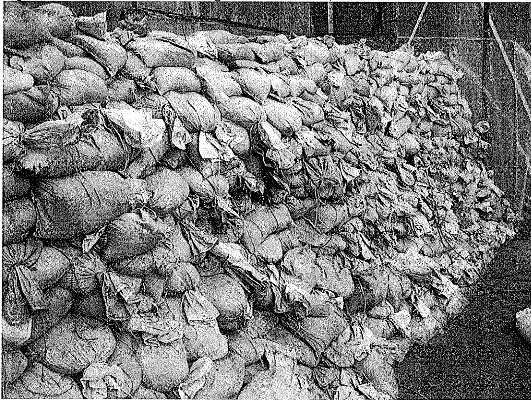
Figure 5.73 – Dike E Ready for Loading, View to the East.
