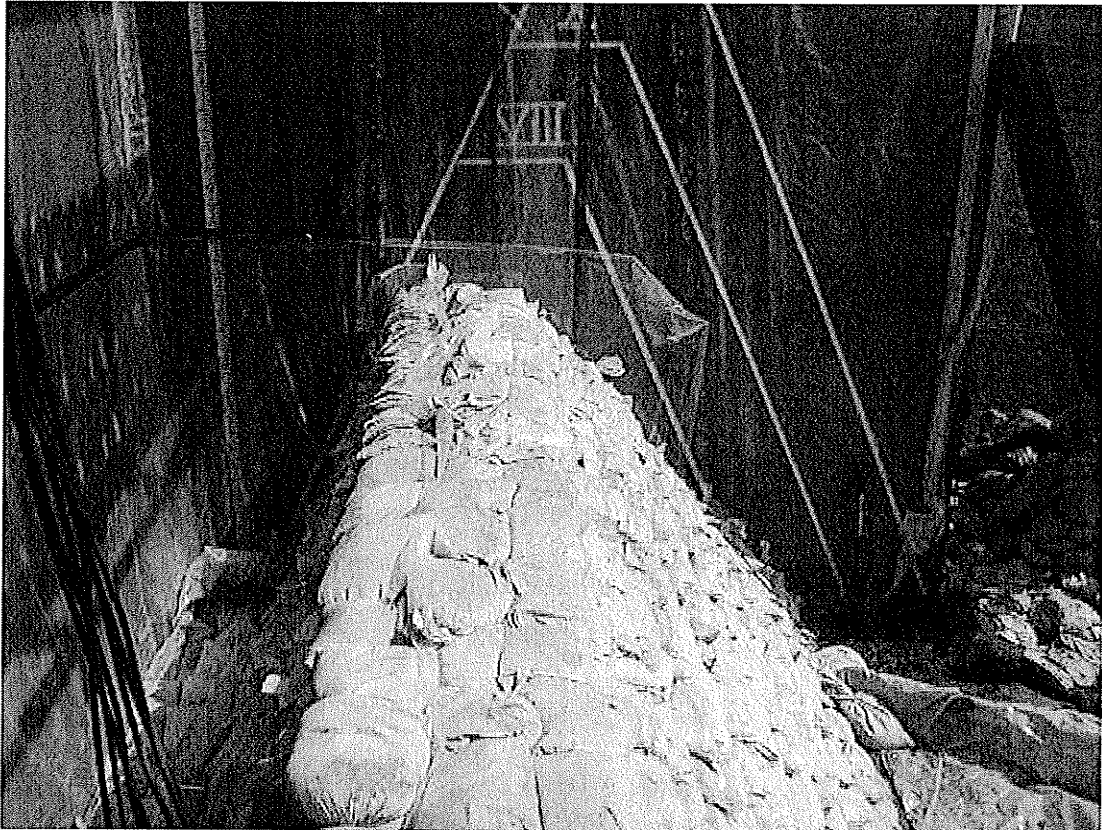
Figure 5.58 – Dike D1 Ready for Loading, View to the East.
