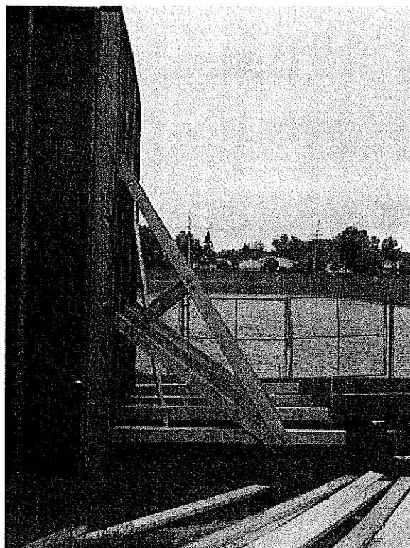
Figure 4.8 – East and West Truss bracing systems under construction (view to the South).
