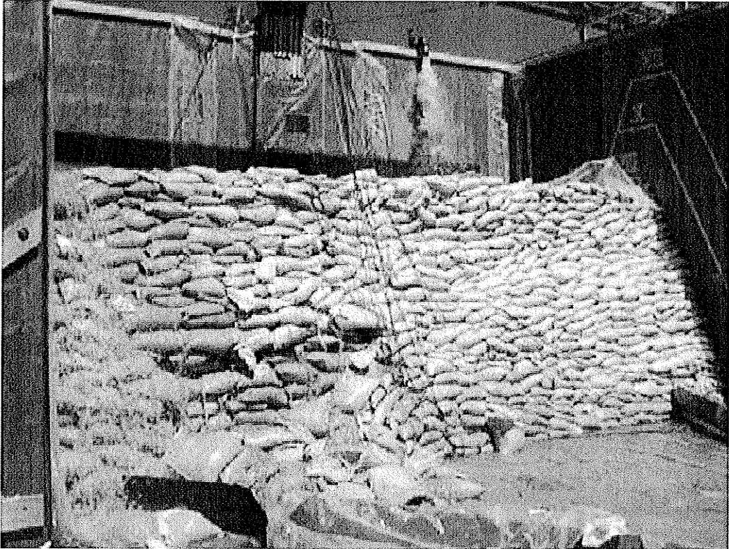
Figure 5.7 – Dike A2 Failing at Overtop Loading.
