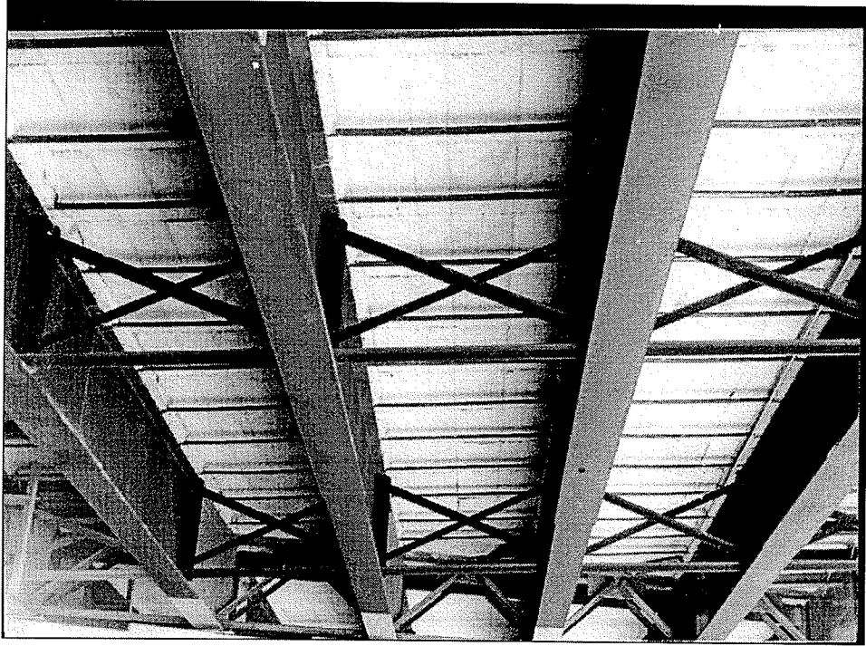
Fig. 2.4(b): Bottom view of Salmon River Bridge
