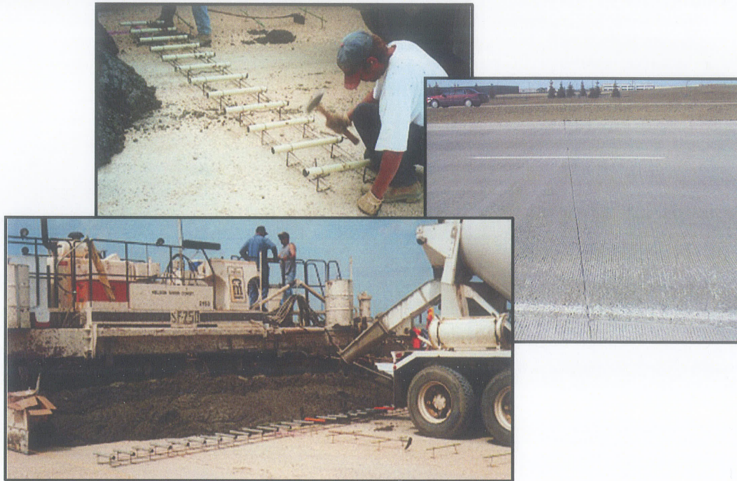
Figure 2.9: Bishop Grandin Field Application with GFRP dowels
