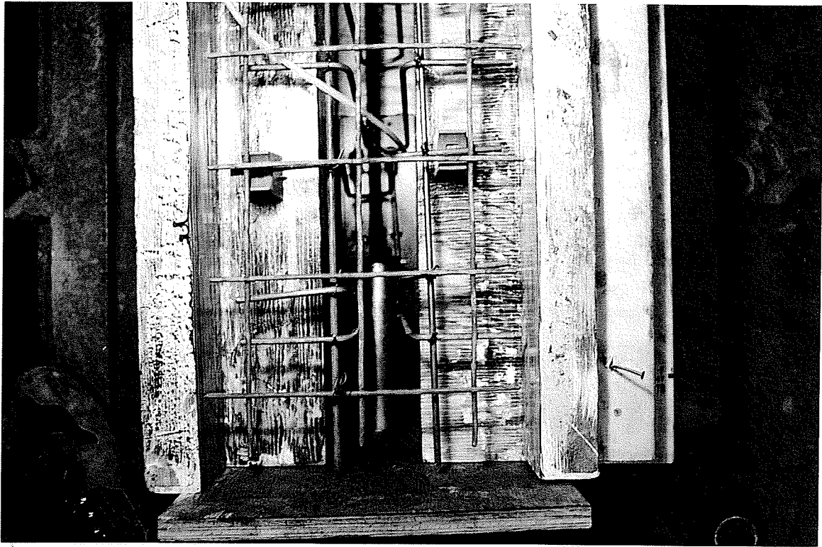
Figure 3.9 Reinforcement at End of Beam
