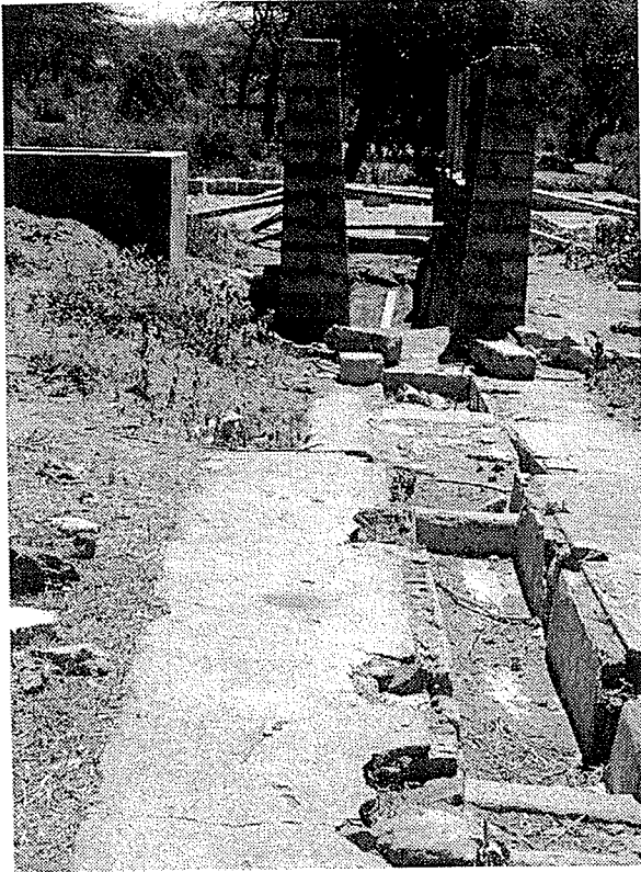
Cattle dip construction is in it's initial stages of construction - August 1999
