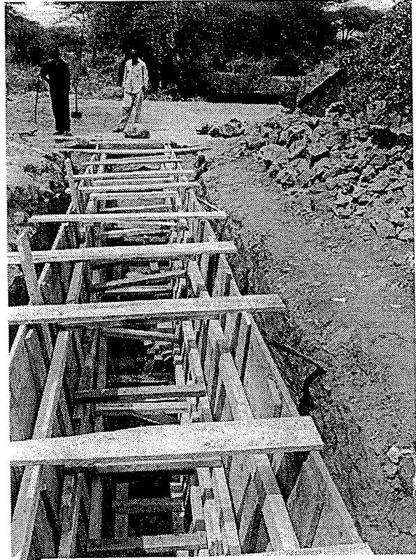
Pit for the cattle dip is excavated during initial stages of construction—August 1999
