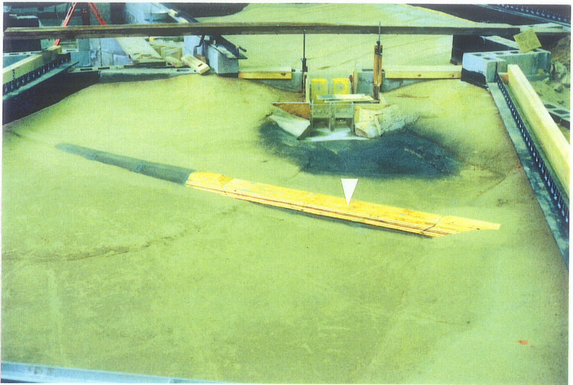
Figure 4.5 Downstream cofferdam constructed with wood and concrete modules for easy adjustments to excavation widths and elevations.
