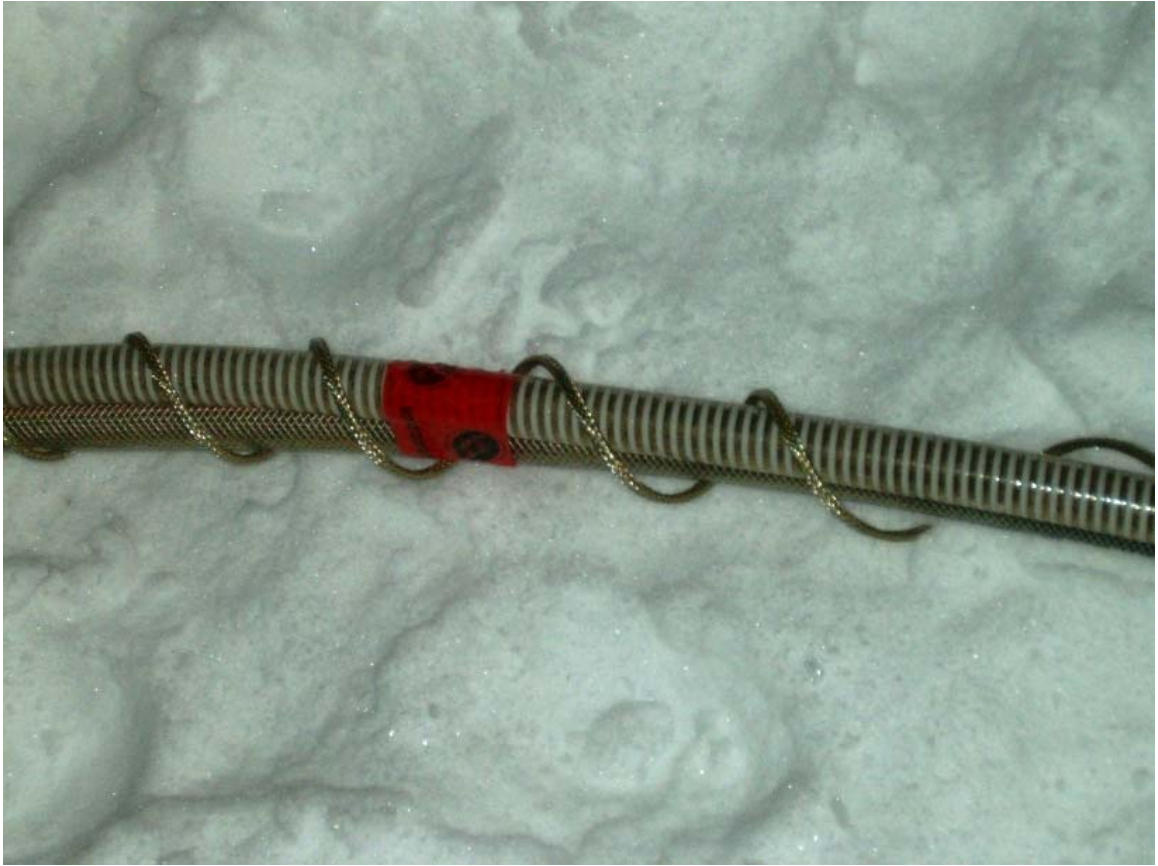
Figure 21: Heat tracing for feed water piping
