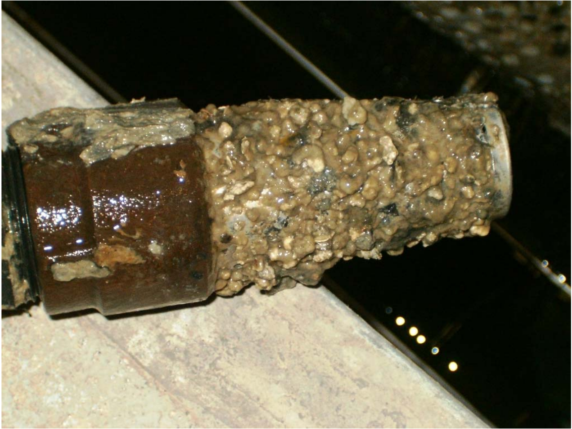
Figure 18: Plugged screen on foot valve.
