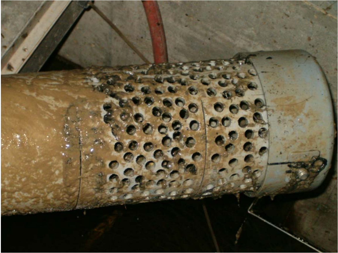
Figure 19: Guard screen for foot valve
