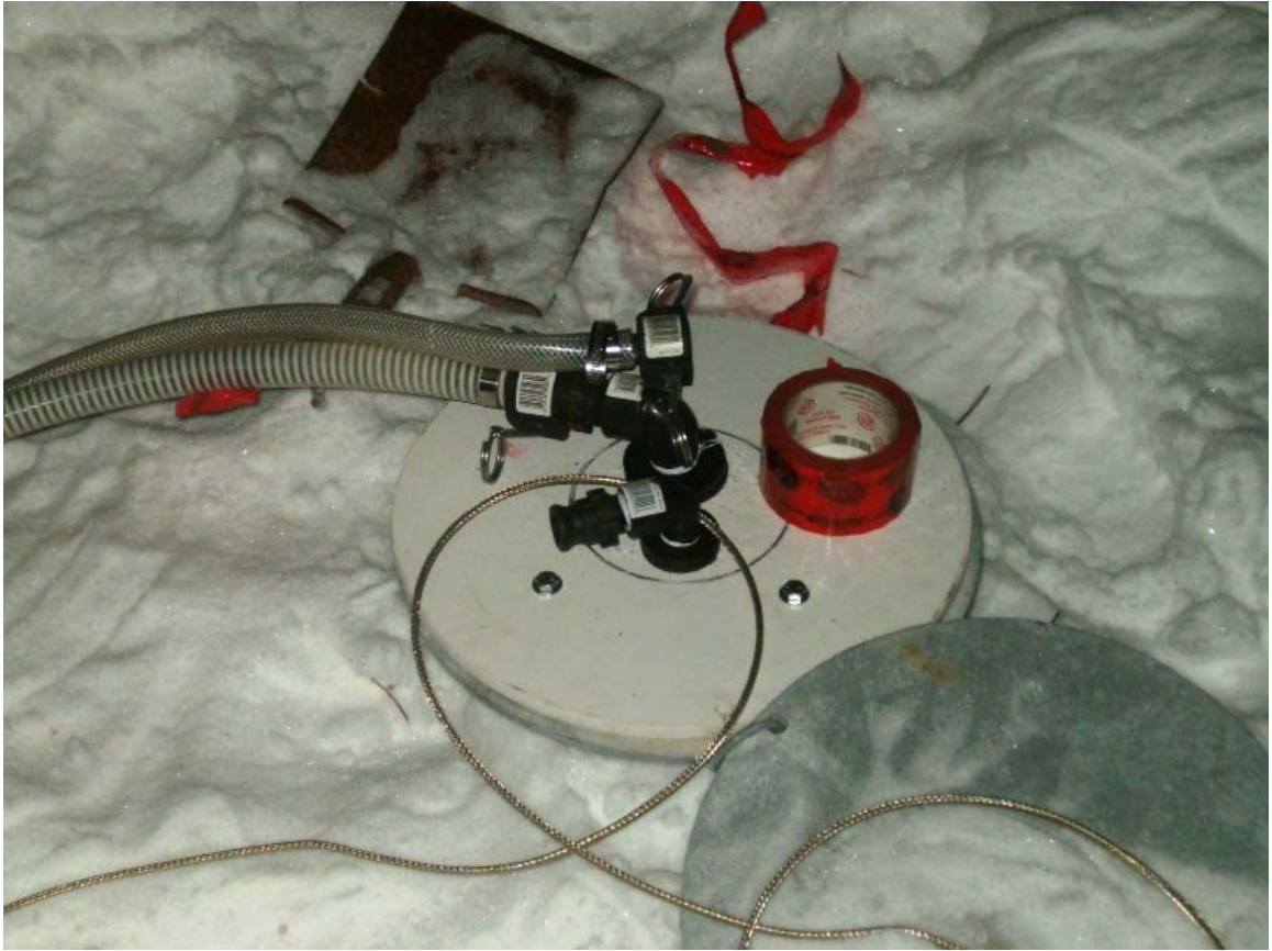
Figure 22: Heat tracing on raw wastewater cap
