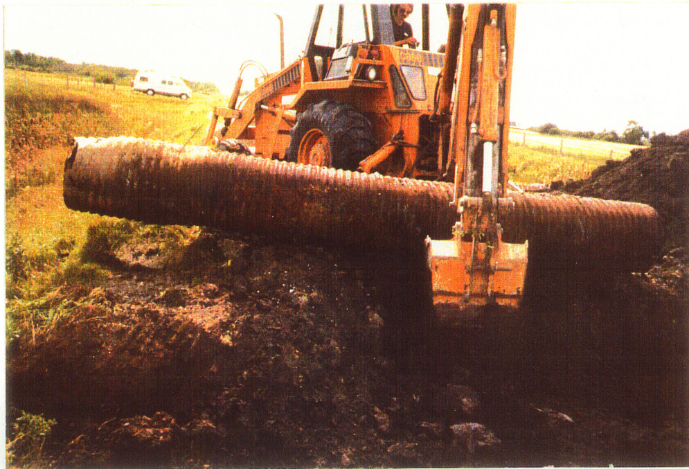
Figure 3.0 Field investigation: Photographs of culvert site near Harding, Manitoba
