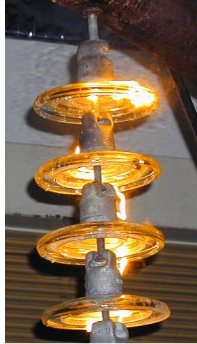
Figure 2.4: Pollution Flashover. Adopted with modification from [6]. Photo ©2001 Stellenbosch University High Voltage Laboratory. Used by Permission.
