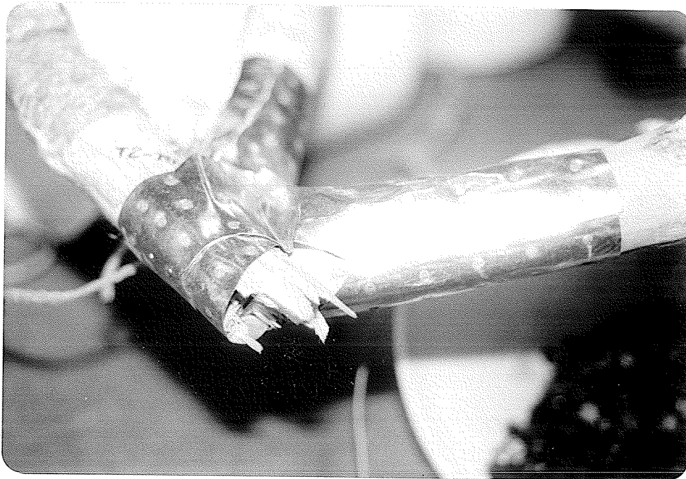
Fig. 5-2: Joint B - Truss T2, Post Collapse
