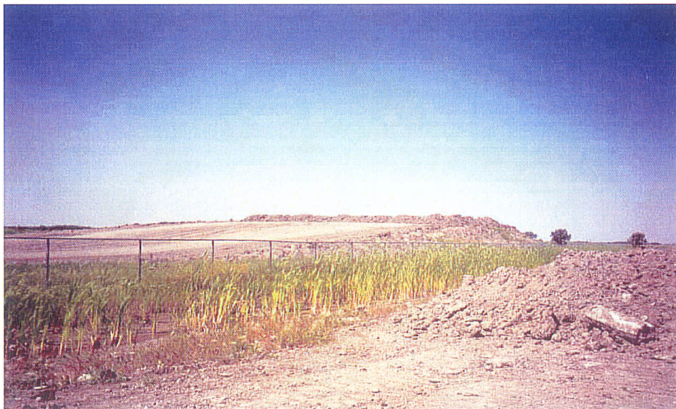
Figure 2.2 Petro-Canada Soil Recycling Facility. Remediated soil is stored until it is used as a backfill material on an industrial site.
