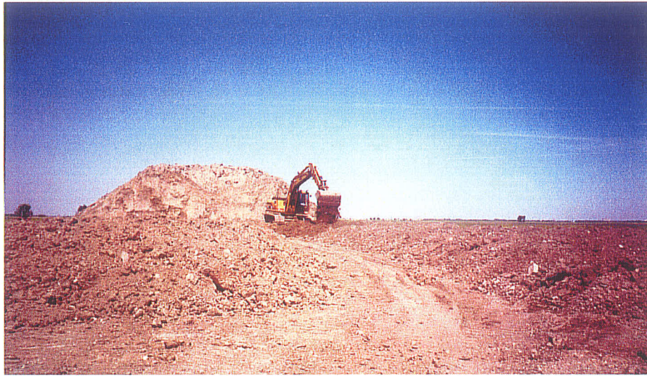
Figure 2.1 Petro-Canada Soil Recycling Facility. The backhoe is aerating the soil to promote aerobic biodegradation and volatilization.
