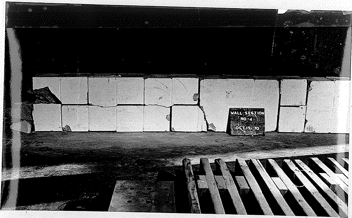
WALL SECTION 4 AT FAILURE
