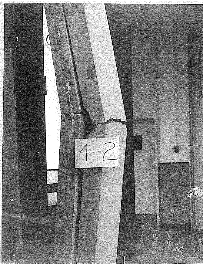
Plate No. 21. Showing panel 4 - 2 at failure.
