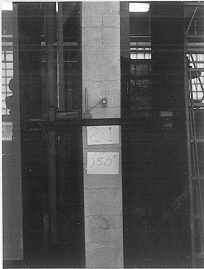
Plate No. 33. Showing panel 2 - 1 during test.
