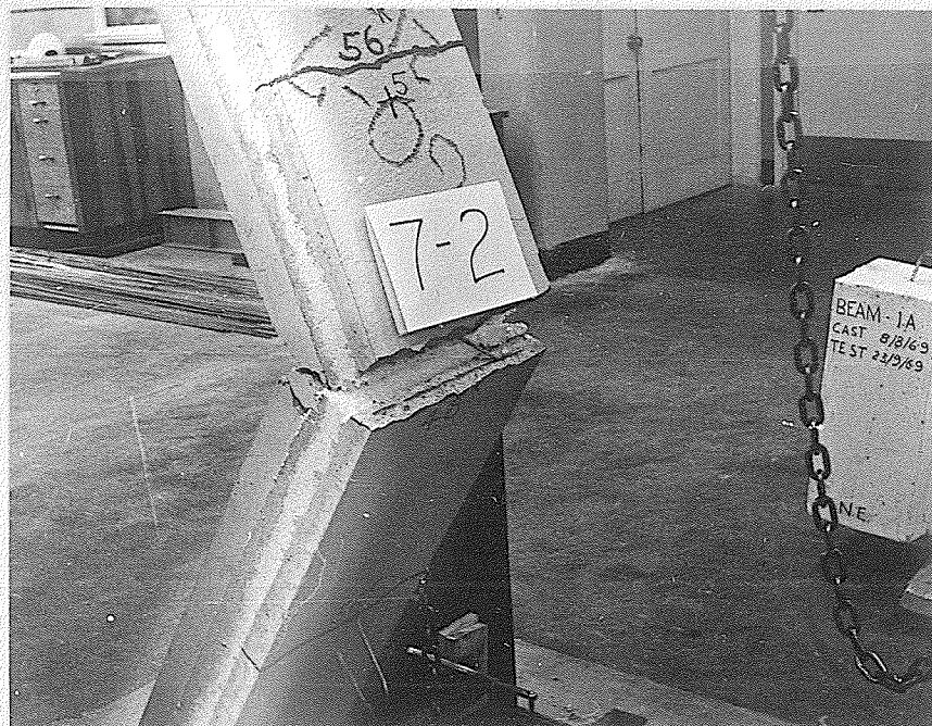
Plate No. 18. Showing panel 7 - 2 at failure.
