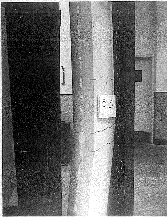
Plate No. 13. Showing panel 8 - 3 at failure.
