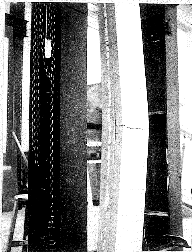
Plate No. 6. Showing panel 9 - 2 at failure.
