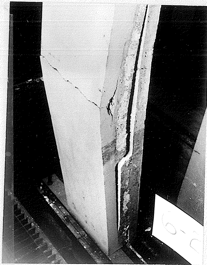
Plate No. 23. Showing panel 6 - 2 at failure.
