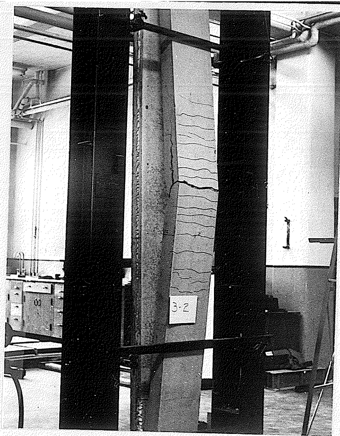
Plate No. 27. Showing panel 3 - 2 at failure.
