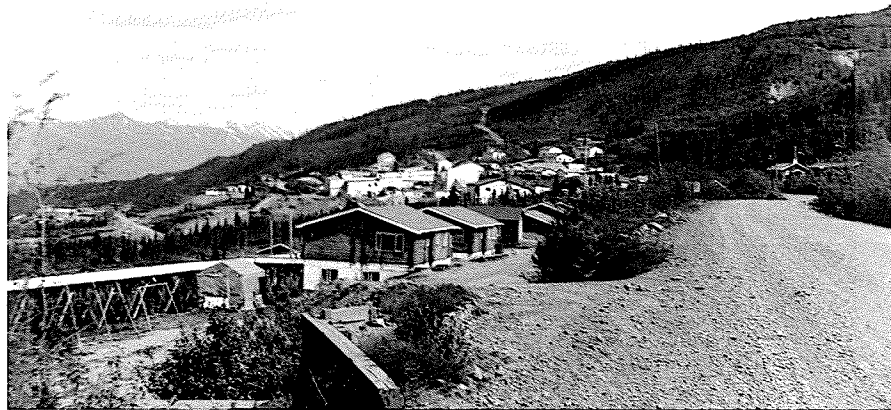
Plate 5: Elsa. As illustrated here Elsa, currently the most prosperous community in the Mayo group, is terraced into a hillside and aligned along the Mayo-Elsa road. In the foreground (left of center) some of the settlement's newer dwellings are to be seen, whilst to the left of these part of the above-surface water conveyance system can be observed.
