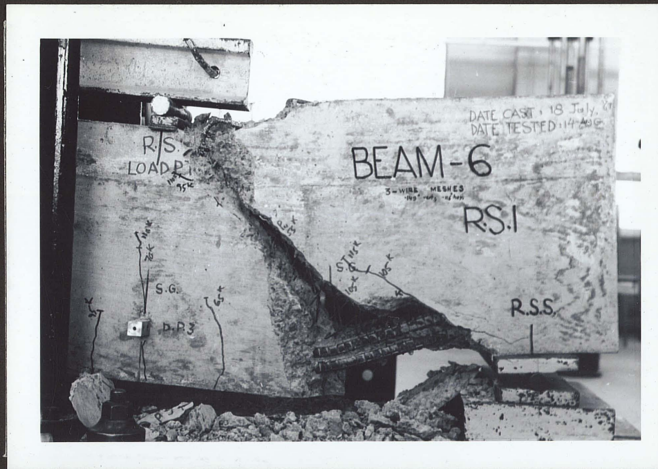
FIG. 71 - Beam 6: Side R.S.1 on Further Loading After Failure
