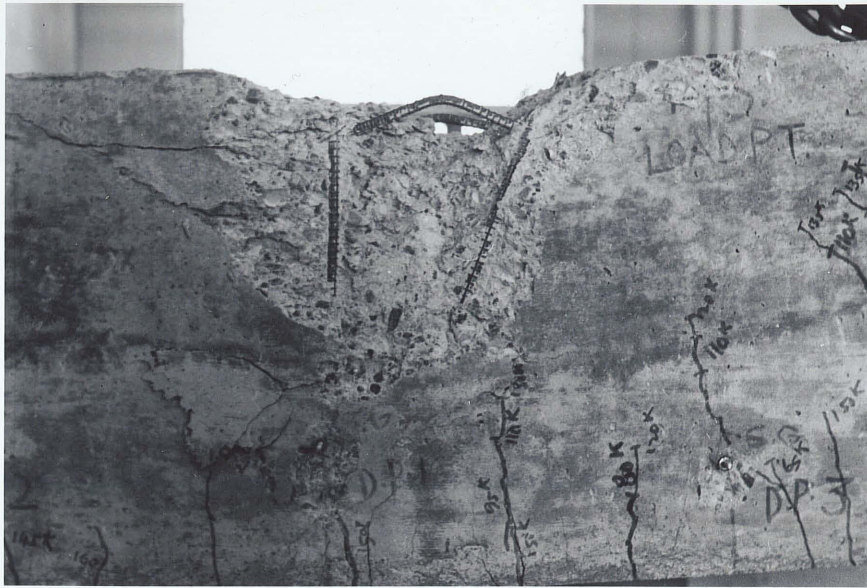
FIG. 65 - Close View of Cracked Portion in Beam 5 (side L.S.1 - R.S.1)
