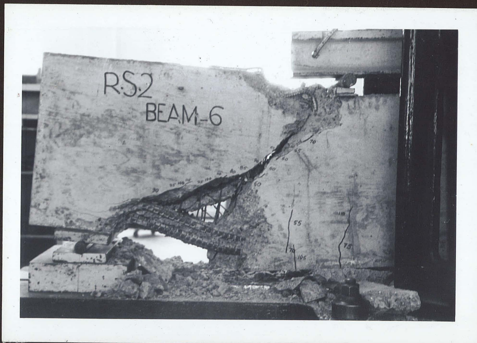
FIG. 73 - Beam 6: side R.S.2 on Further Loading after Failure
