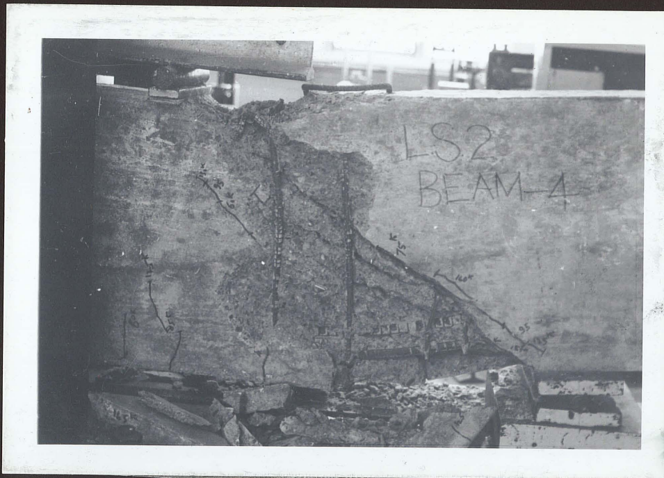
FIG. 59 - Beam 4 (side L.S.2) after Complete Failure
