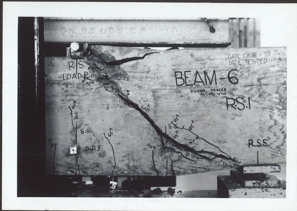
FIG. 70 - Beam 6: Close view of side R.S.1 after Failure
