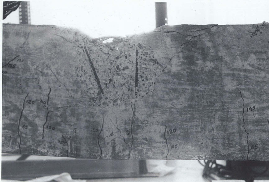
FIG. 66 - Close View of Cracked Portion in Beam 5 (side R.S.2 - L.S.2)
