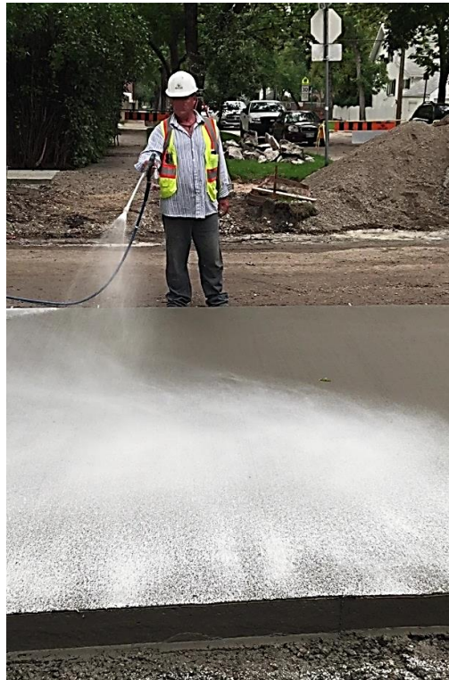
Figure 2.1- Applying curing compound on concrete pavement.
