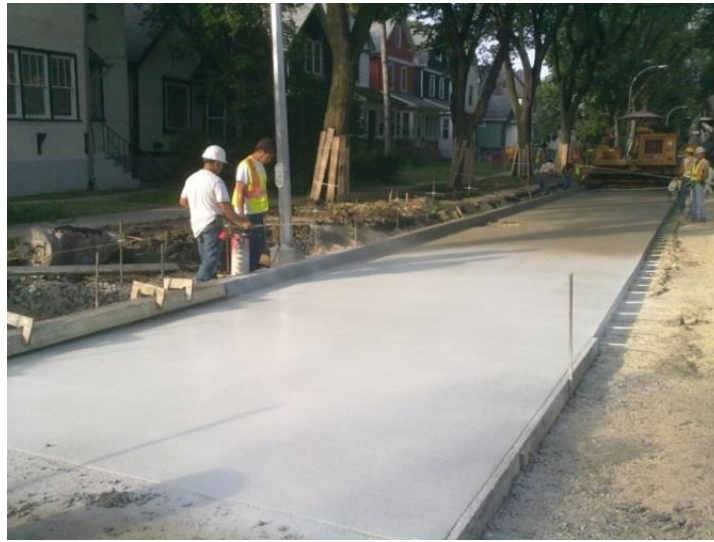
Figure 3.1- Casting, finishing and curing procedures of field pavement sections.
