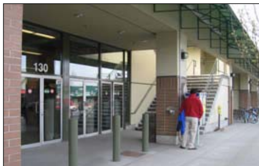
Figure 4.24 Stairwell and elevator at the front entrance leading to the roof-top parking lot.
