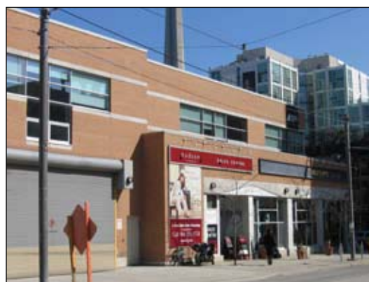
Figure 4.54 Pedestrian access from the parking lot to the front entrance of the building is safe for customers.
