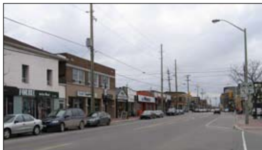
Figure 4.95 One and two-storey buildings on small lots with narrow storefronts.
