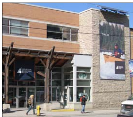
Figure 4.58 A large picture (below the photovoltaic panels) displaying MEC products and activities helps to identify the retailer.
