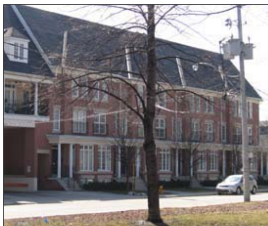
Figure 4.37 Three-storey rowhousing next to a park in the King-Spadina district.
