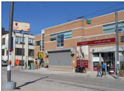
Figure 4.50 Even the side of the MEC building is interesting for pedestrians. The loading bay and parking lot entrance is located along this wall, but is not an eyesore!
