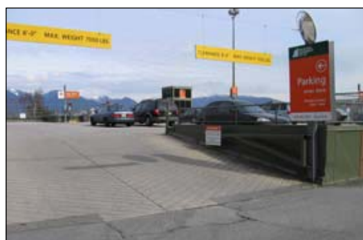
Figure 4.21 The ramp at the back of the site leading to the roof-top parking lot.
