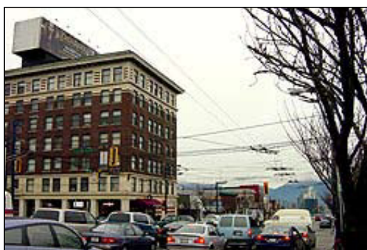
Figure 4.6 Character building at Broadway and Main Street.
