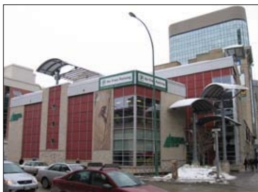
Figure 4.137 The combination of materials, textures and images on the side of the building enhances the visual appeal.
