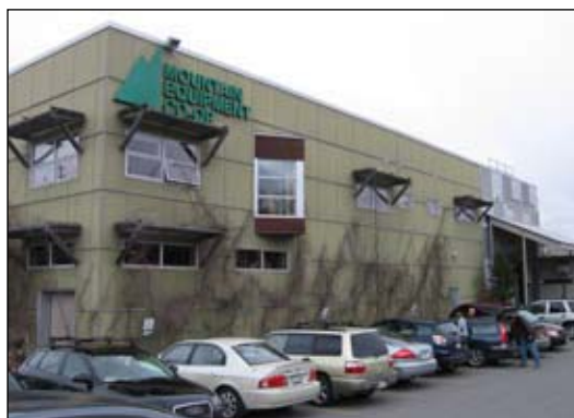
Figure 4.116 The on-site parking is located at the side and rear of the building.
