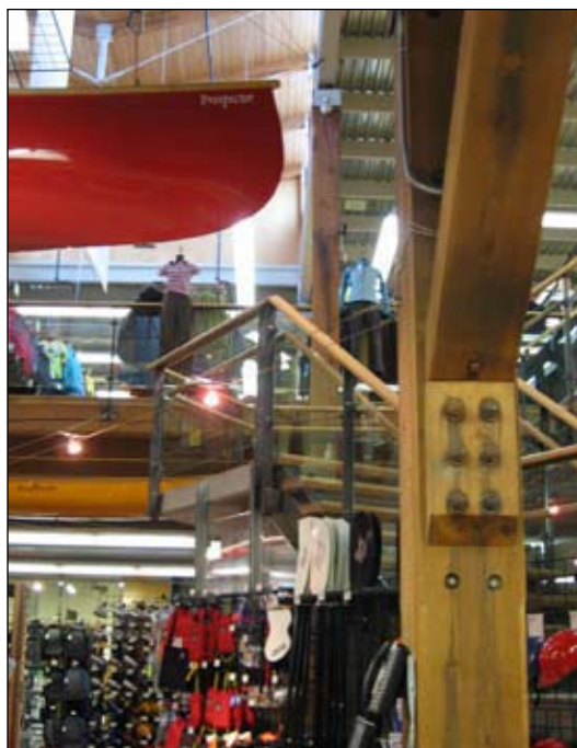
Figure 4.105 Many materials used in the construction of the Ottawa store were reused or recycled.
