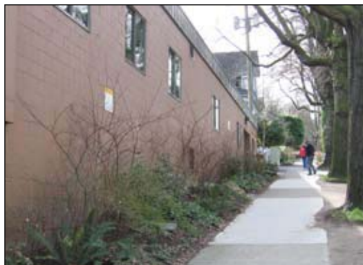
Figure 4.20 Exterior of the building on the west side is landscaped to reduce site runoff and increase the aesthetics.
