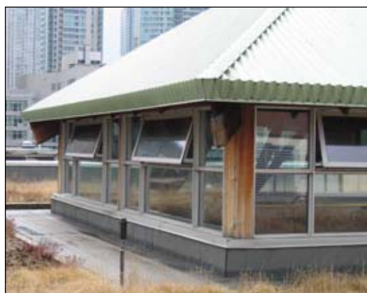
Figure 4.63 Windows are mechanically opened and closed to control indoor temperature.
