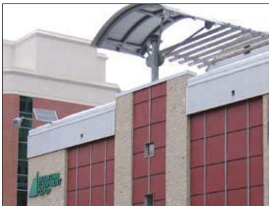
Figure 4.142 The solar panel which powers the irrigation pump is just barely visible on the roof.
