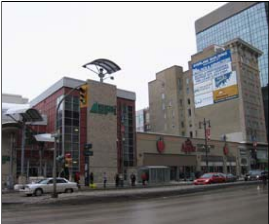
Figure 4.131 Scale of buildings on the block range from one to fifteen storeys high.
