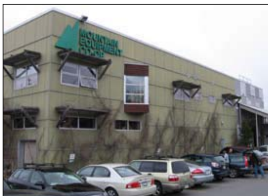
Figure 4.108 Window shades and vines reduce cooling needs in the summer heat.
