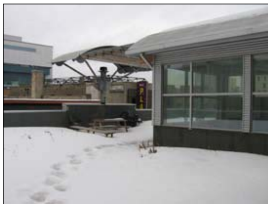
Figure 4.141 The roof-top garden reduces stormwater runoff, naturally cools the building and provides a green space for building workers.
