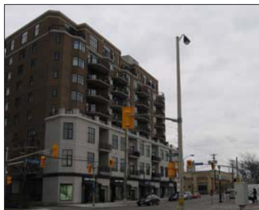
Figure 4.71 New apartment-condominium building development on Richmond Road.
