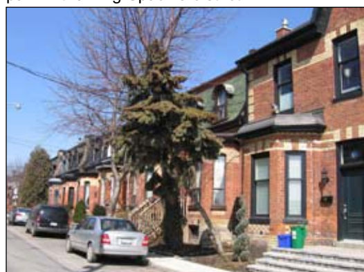
Figure 4.38 Two-storey rowhousing next to a park in the King-Spadina district.
