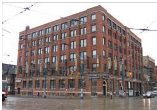
Figure 4.36 Character of the warehouse buildings in the King-Spadina district, looking west on King Street.
