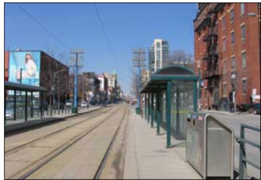
Figure 4.33 A major street car transit station on Spadina at King Street.
