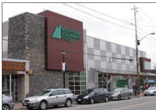
Figure 4.110 Facade of the Ottawa MEC store facing Richmond Road.
