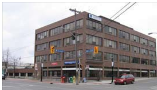
Figure 4.101 An office building and associated parking garage sit vacant.
