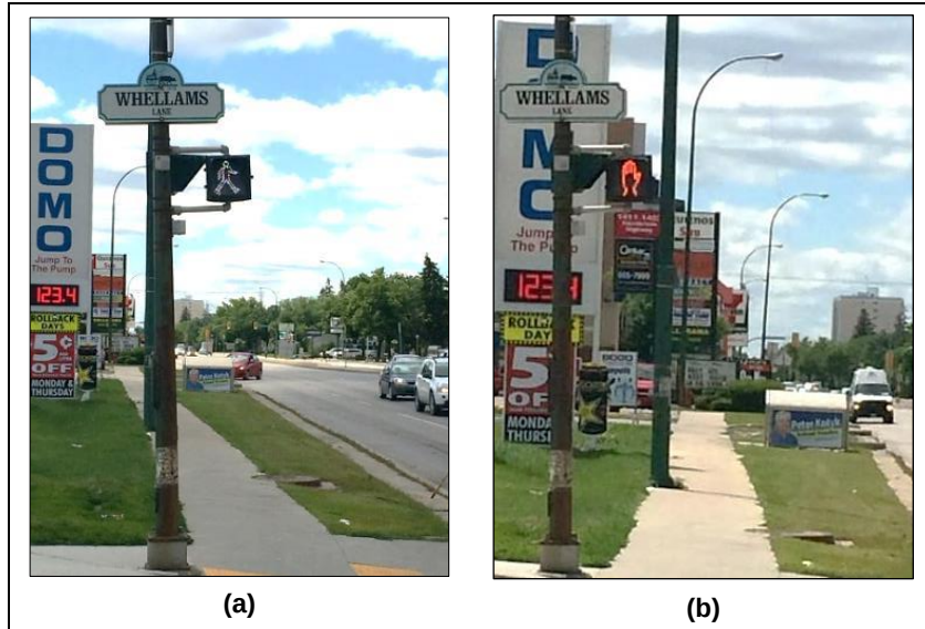
Figure A44: Typical pedestrian signal displays in Canada: (a) walking pedestrian display for WALK interval; (b) hand display for DON'T WALK interval (flashes during Flashing DON'T WALK interval)
