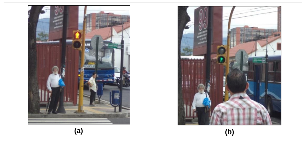
Figure A61: Typical pedestrian signal displays in Costa Rica: (a) Standing red person for DON'T WALK interval; (b) Walking green person for WALK interval (flashes during Flashing WALK interval)
