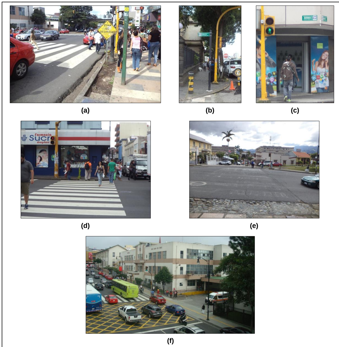
Figure 15: Signage and pavement markings: (a) Zona de Seguridad (Safety Zone) sign; (b) Post-mounted street sign; (c) Wall-mounted street sign; (d) Zebra markings in good condition; (e) Zebra markings in poor condition; (f) Stop line set back to accommodate ambulance entrance to hospital
