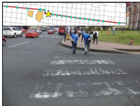
Figure 7: Zebra markings on the minor street approach at Site 7
