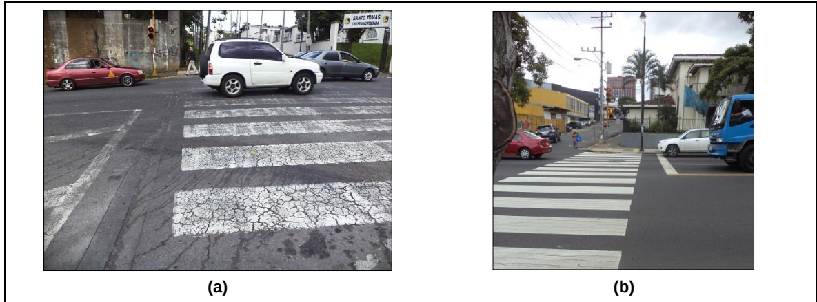
Figure 11: Surface condition: (a) Acceptable; (b) Good
