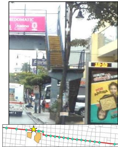
Figure 5: Stair access onto pedestrian overpass
