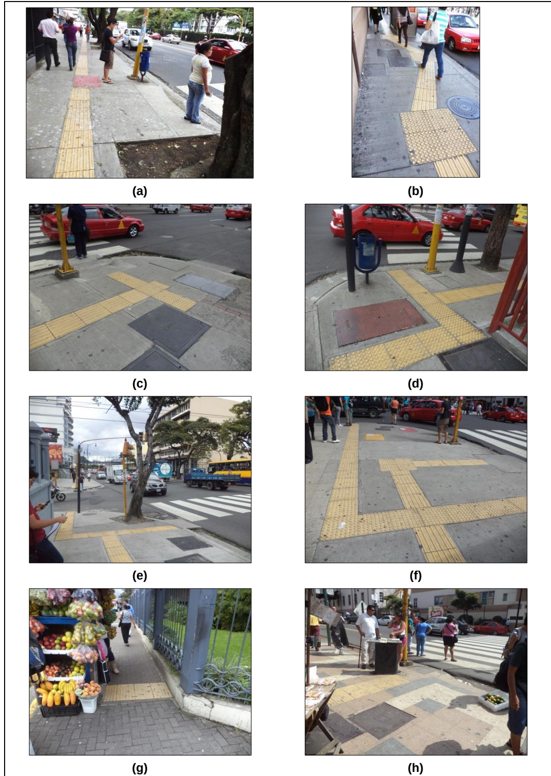
Figure 20: Tactile markings: (a) Directional surface on sidewalk broken by grate; (b) Directional surface on sidewalk changing direction for grate; (c) Incomplete squared off application at terminal due to grates; (d) Crosswalk located outside of squared off area at terminal, obstacles not marked; (e) Crosswalk located inside of squared off area at terminal, transverse strip of detectable warnings terminates at curb ramp, obstacles not marked; (f) Directional surface leads to curb ramp at terminal with squared off application; (g) Vendor set up over transverse strip of detectable warnings at terminal; (h) Transverse strip of detectable warnings at terminal;
