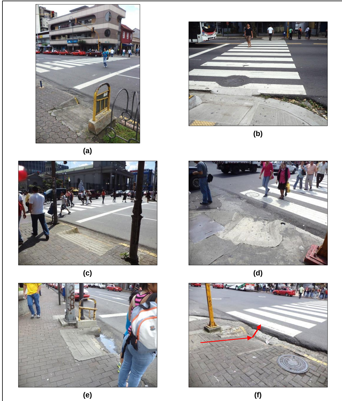
Figure 19: Curb ramps: (a) Ramp with handrail located outside of zebra markings; (b) Aligned ramps and with cut asphalt overlay for accessible upward grade; (c) Ramp located outside of zebra markings and directed into traffic lanes; (d) Ramp directed to the centre of the intersection with narrow ramp width; (e) Gap between bottom of curb ramp and crosswalk/roadway with ponding; (f) Upward grade between bottom of ramp and crosswalk/roadway caused by asphalt overlay
