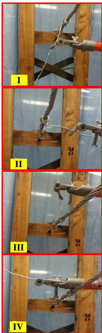
(a) Twisting a tie wire (Task A)
