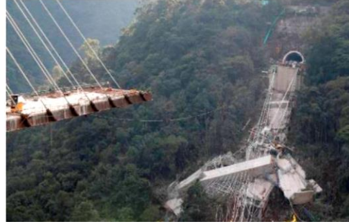
Figure 5. Bridge failures due to design errors. (a) Defects in design theory. (b) Design mistake [12]
