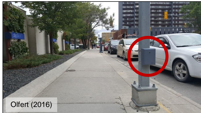
Figure 3: Eco-Counter PYRO-Box Installation
