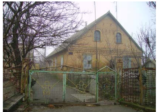
A-3 A typical Mennonite home still standing in many villages, constructed late 19 th century, Ukraine, 2005, Personal Photographs
