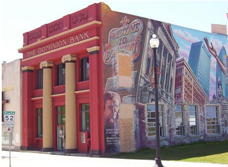
Figure 11a: Dominion Bank Building before the addition of Bridgman Collaborative Architecture. Retrieved from: http://westenddumplings.blogspot.ca/2008/06/winnipegs-main-street-redevelopment.html
