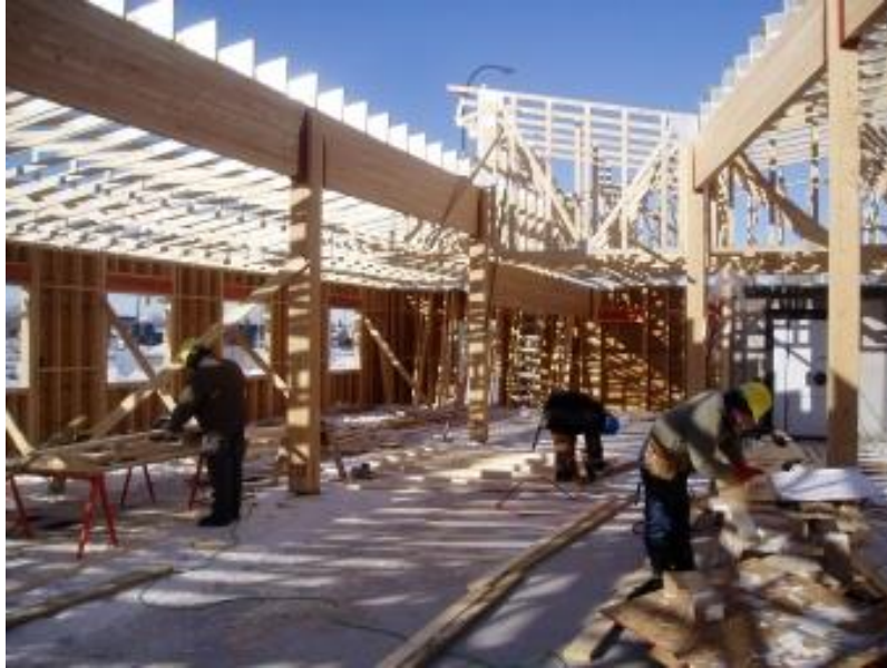
Figure 10a: Assiniboine Credit Union Rivergrove Branch under construction.
