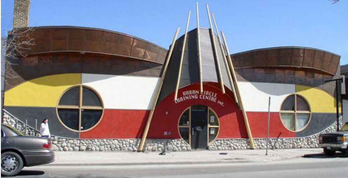
Figure 9: Completed structure of Urban Circle Training Centre at Selkirk Avenue.
