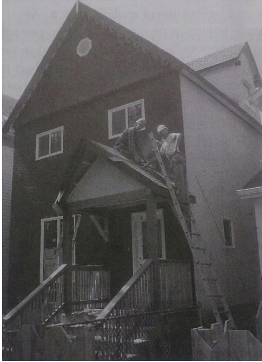
Figure 8a: ICR's renovation work at Spence neighbourhood. Retrieved from: Donkervoort, 2013, p. 5.
