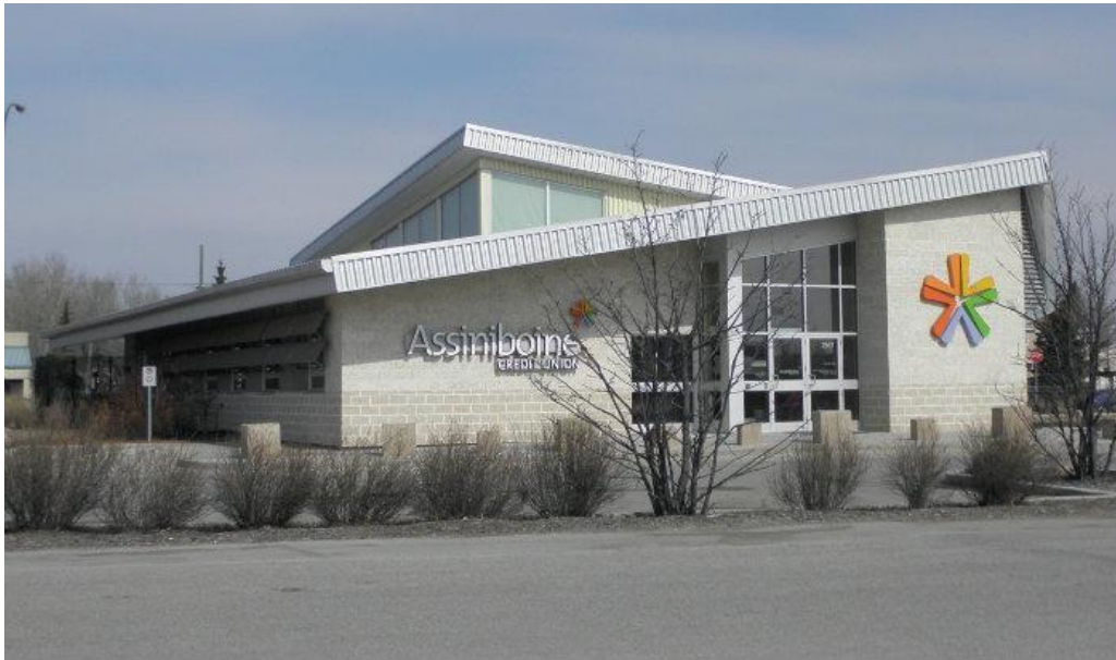
Figure 10b: Completed structure of Assiniboine Credit Union Rivergrove Branch.
