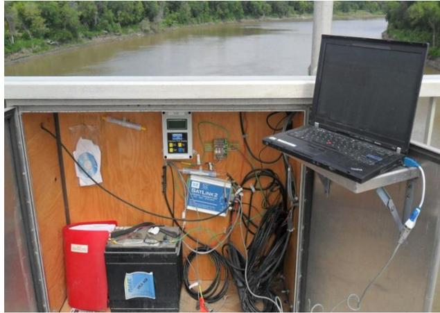
Figure 3.1: SPB water level recording station
