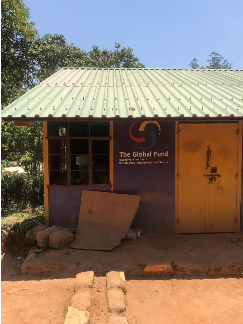
Figure 10. A mural of the Global Fund on the wall of a building that is locked and seemingly empty. It seems especially forlorn since I took the picture in 2017 while all nurses and clinical officers were on strike, protesting against low salaries, effectively shutting down services at almost all health facilities.
