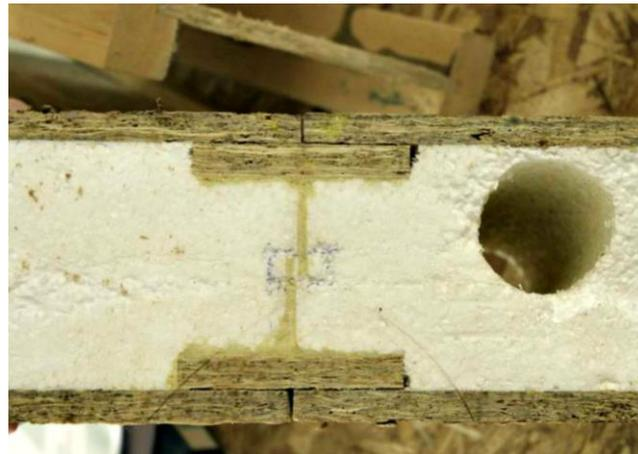
Figure 3-7: A typical spline-glue connection used to connect two Styrofoam foam core panels together (Fine Homebuilding, 2006)
