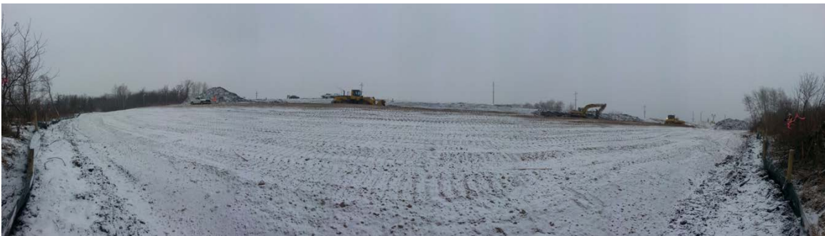
Photo 24 – Fill Placement for Upper Berm
