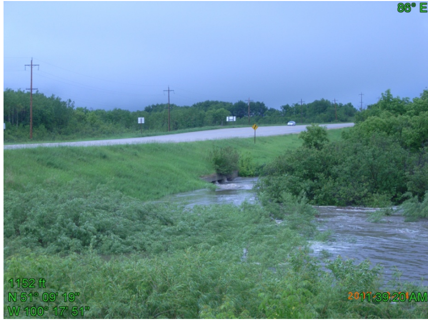
Figure 3.23 – Triple Box Culvert, PTH 5 East of Slide Area (June, 2013)
