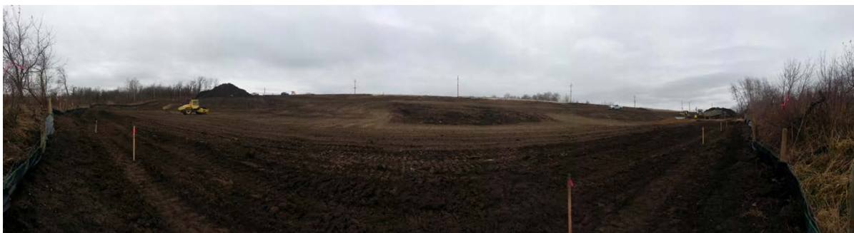
Photo 18 – Grading at Toe of Lower Berm Prior to Fill Placement
