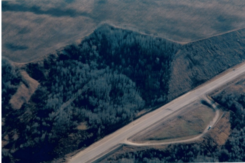
Figure 2.1 – Oblique View of PTH 83 at Shell River Slide Area (Note slump block in backslope)
