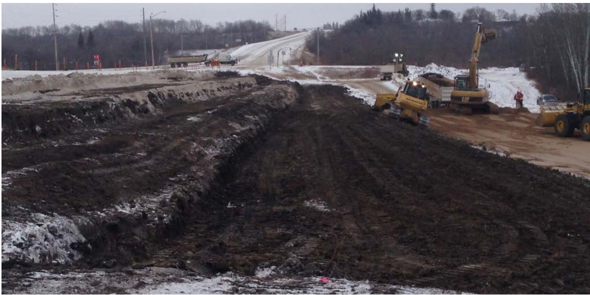
Photo 23 – Bench Cuts Prior to Fill Placement for Upper Berm
