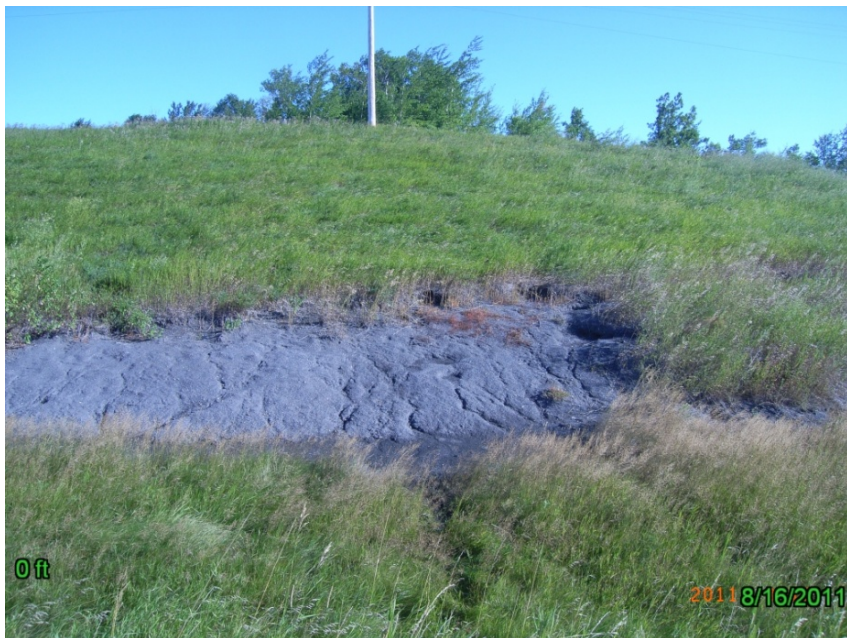
Figure 3.2 – Exposed Weathered Clay Shale in Backslope
