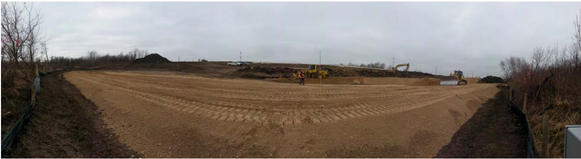
Photo 20 – Grading of Lower Berm
