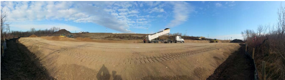
Photo 21 – Fill Placement on Lower Berm
