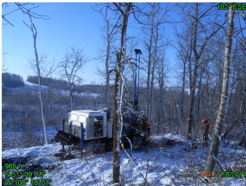
Figure 4.3 – Phase II Drilling, TH2011-05 (November, 2011)
