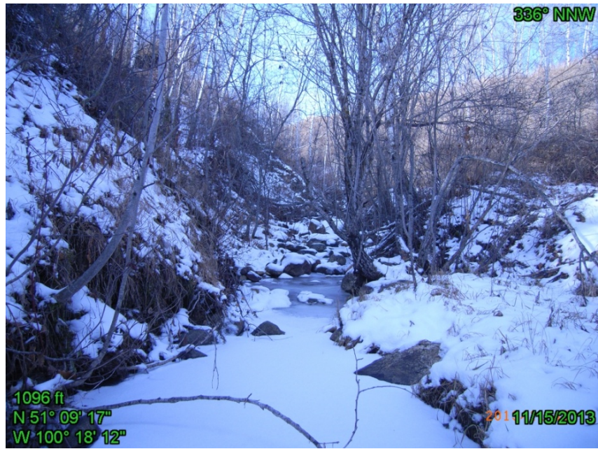
Figure 1.8 – 1965 Drain Eroded into Mineral Creek Valley Wall (North from drain outfall at Mineral Creek)
