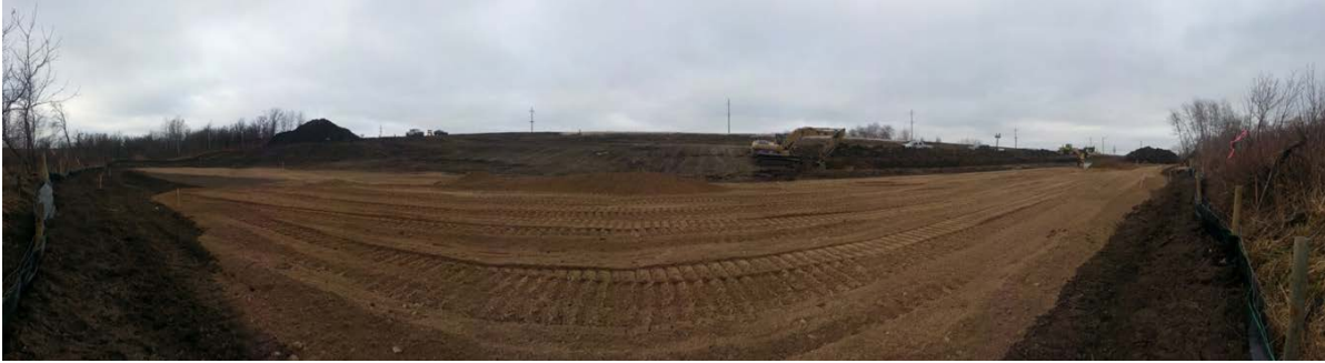
Photo 19 – First Lifts of Lower Berm
