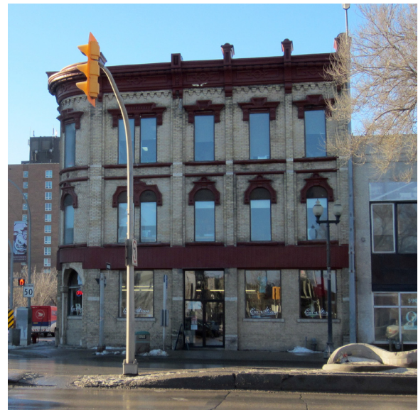
Figure 5.4.2.6 – Maycock Block, West Elevation
