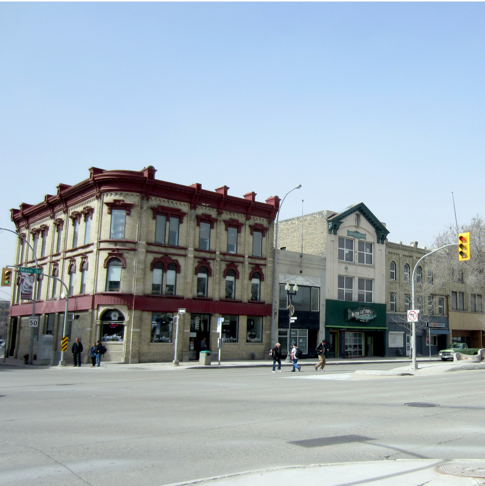
Figure 5.4.2.1 – Maycock Block, existing exterior
