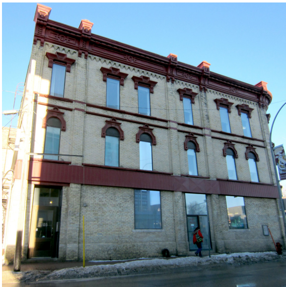
Figure 5.4.2.5 – Maycock Block, North Elevation
