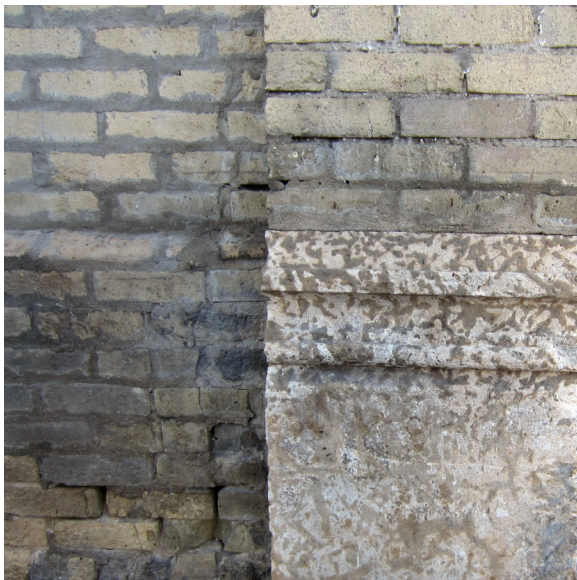
Figure 5.4.2.3 – Maycock Block, Brick Detail
