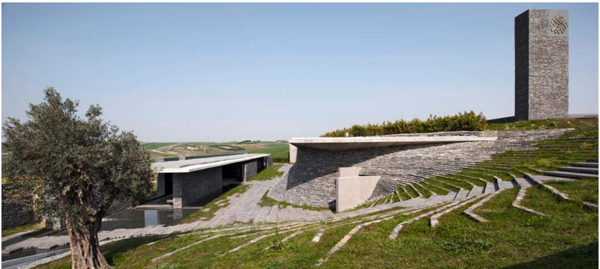
Figure 15. Thomas Mayer (Photographer). (2014). Cascading steps leading to courtyard, [digital photograph], Used with permission obtained September 16, 2015. Purchased September 16, 2015 from http://thomasmayerarchive.de/index.php?!=english .
